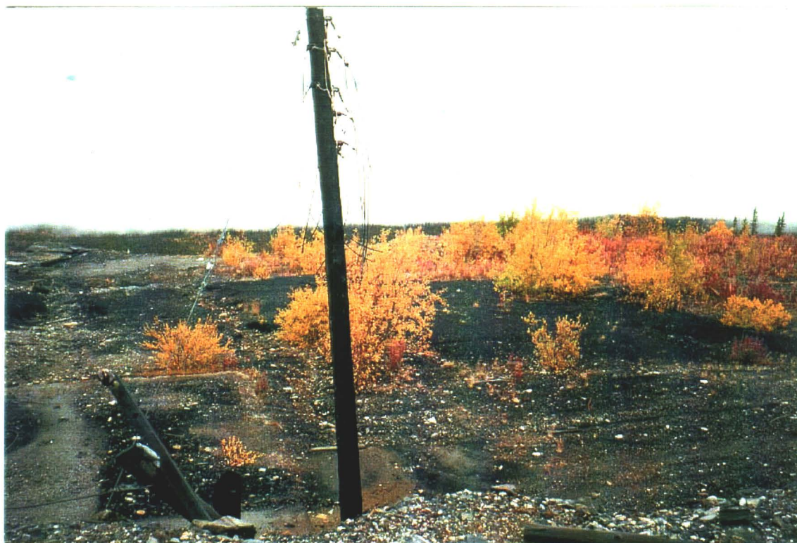
Photo 9-18. Coal piles at site of old steam plant. An edge of the concrete foundation of the plant can be seen on the left side of the photograph.
