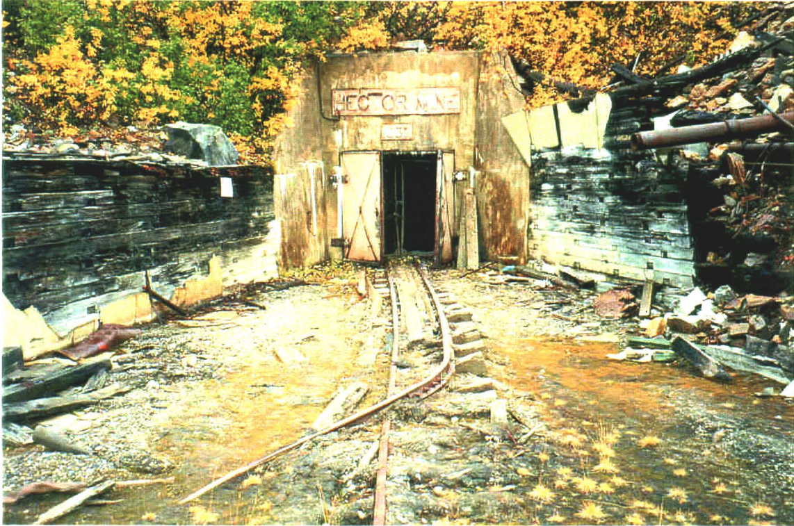
Photo 9-1. Hector Adit, showing the buttressing, old rails and debris.
