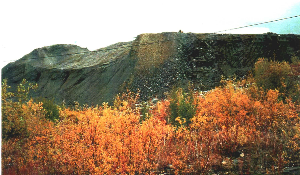
Photo 9-4. Hector dump, looking northwest. Note old wooden buttresses and debris.
