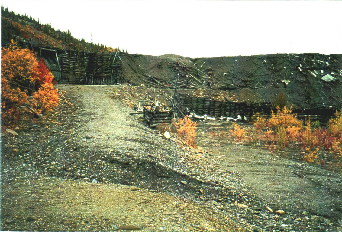
Photo 9-17. Hector dump and loading facility, looking southwest.
