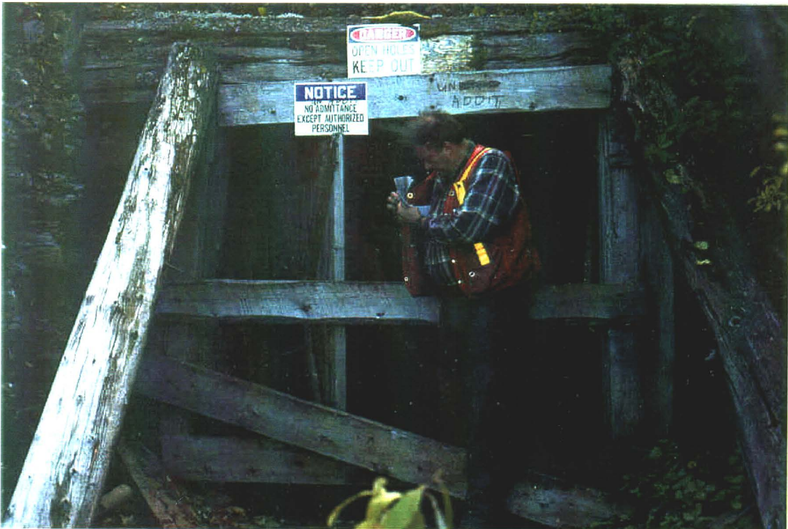
Photo 10-2. UN portal showing wooden debris and open door.
