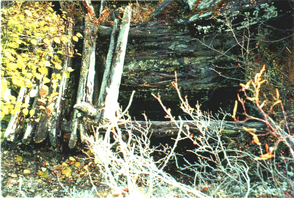
Photo 11-3. Unnamed Shaft. The wood constructing the shaft is rotted and unstable, and the area around the shaft is overgrown.
