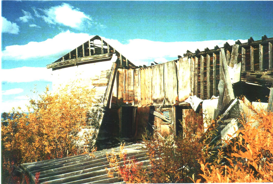
Photo 11-13. Building 11G, showing the remaining walls.
