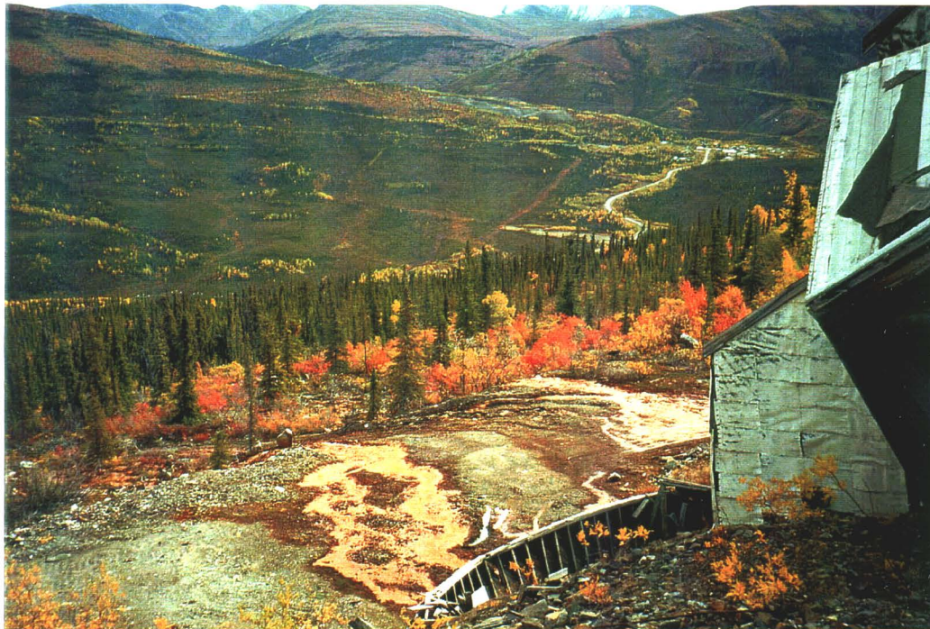
Photo 11-20. Drainage from the 300 level adit as it flows past the Loading Elevator and down below the mine site.
