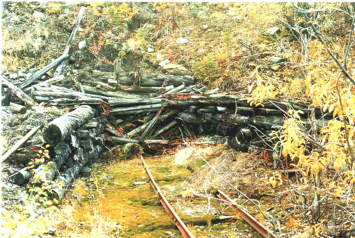
Photo 11-6. Galkeno 100 level adit. Portal is completely collapsed. Note rails exiting adit.
