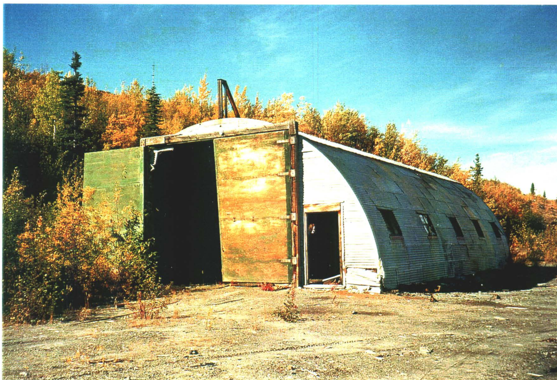
Photo 11-11. Building 11A - Quonset Warehouse, looking northwest. Located near the 300 level adit.
