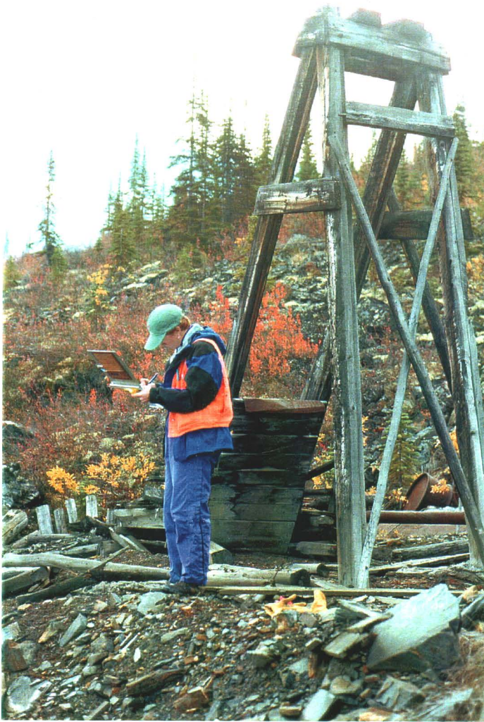
Photo 11-1. McLeod Shaft, looking southeast.
