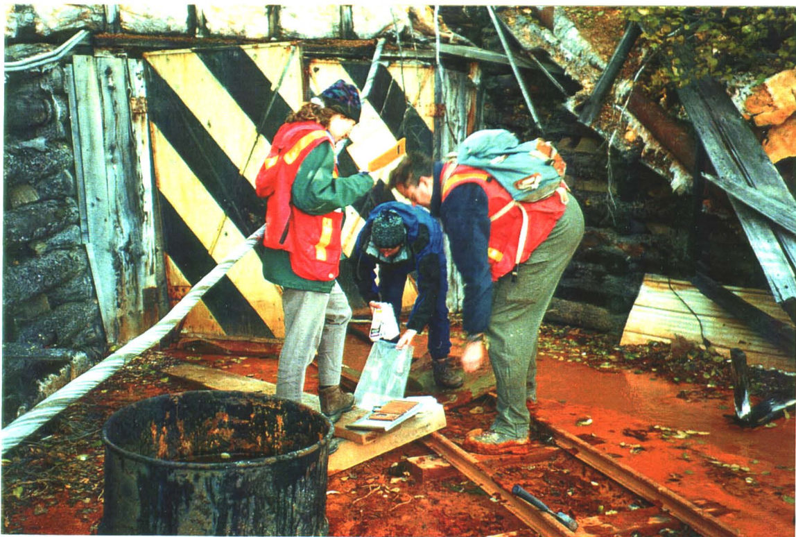
Photo 11-4. Galkeno 300 level adit. Note the iron oxidized (orange) laden water and precipitate. Also note the debris in the area.
