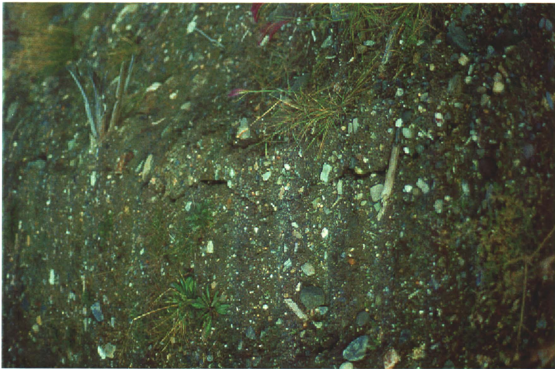
Photo 12-6: Tension cracks in the settling pond retaining wall. (Azimuth 000°)
