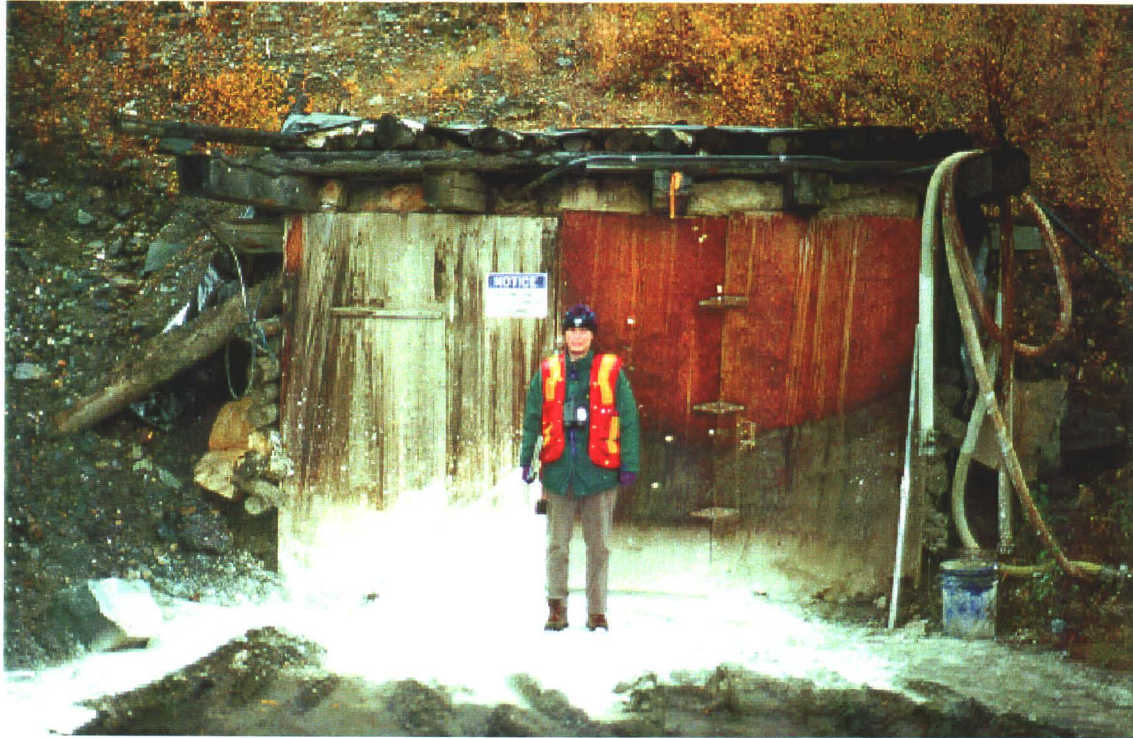
Photo 12-1: Galkeno 900 portal with spilt lime out front, the water treatment facility is located within the adit. (Azimuth 270°)
