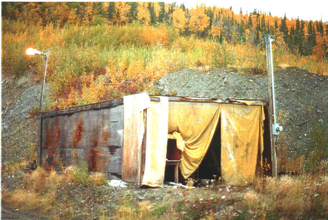
Photo 12-8: Building 12A - a storage building currently in use. (Azimuth 320°)
