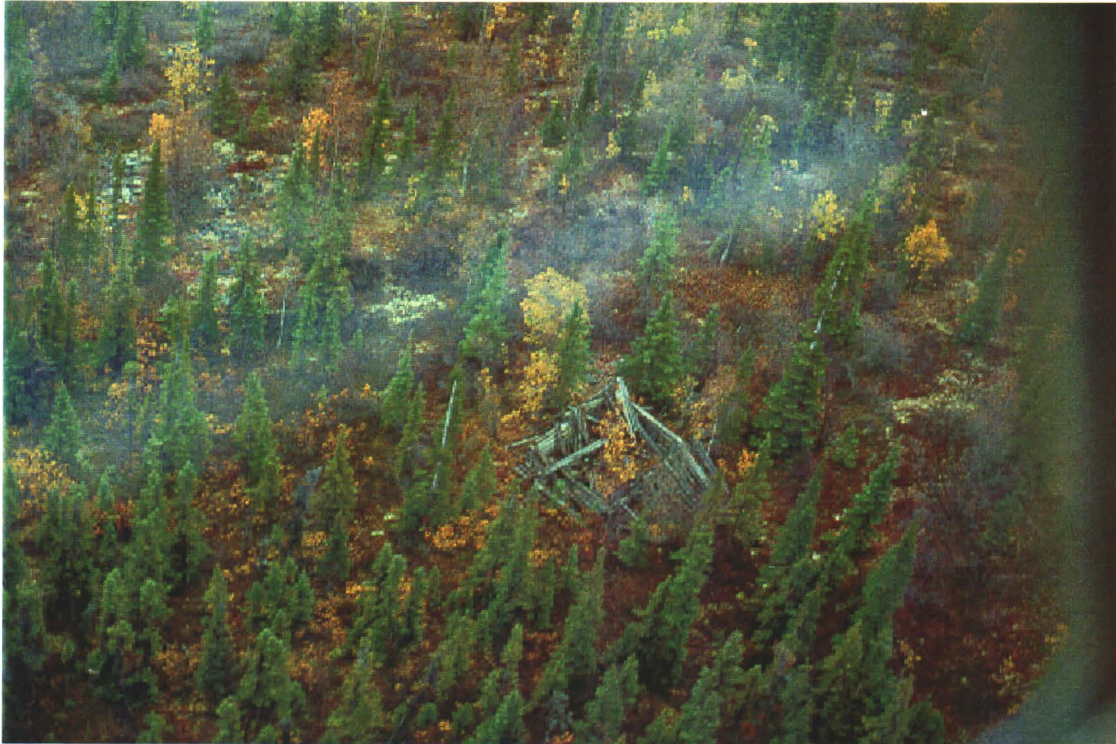
Photo 13-3: Aerial shot of the collapsed log cabin. (Azimuth 260°)
