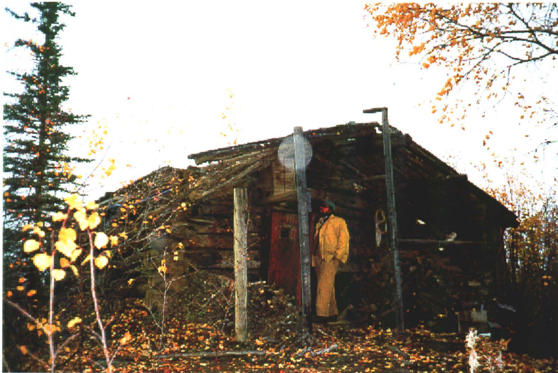
Photo 14-6: Recent cabin (early 1980's); note collapsed sod roof structure. (Azimuth 340°)
