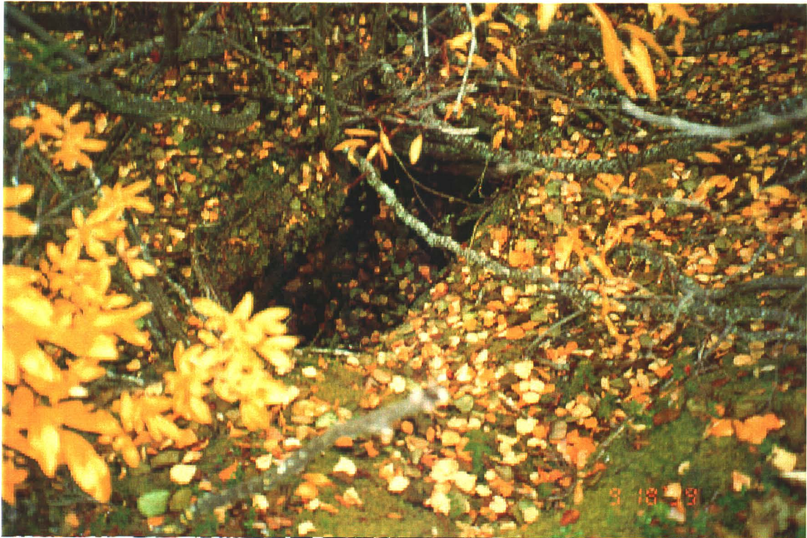
Photo 15-1: Remains of shaft #1. Note water level just below grade.
