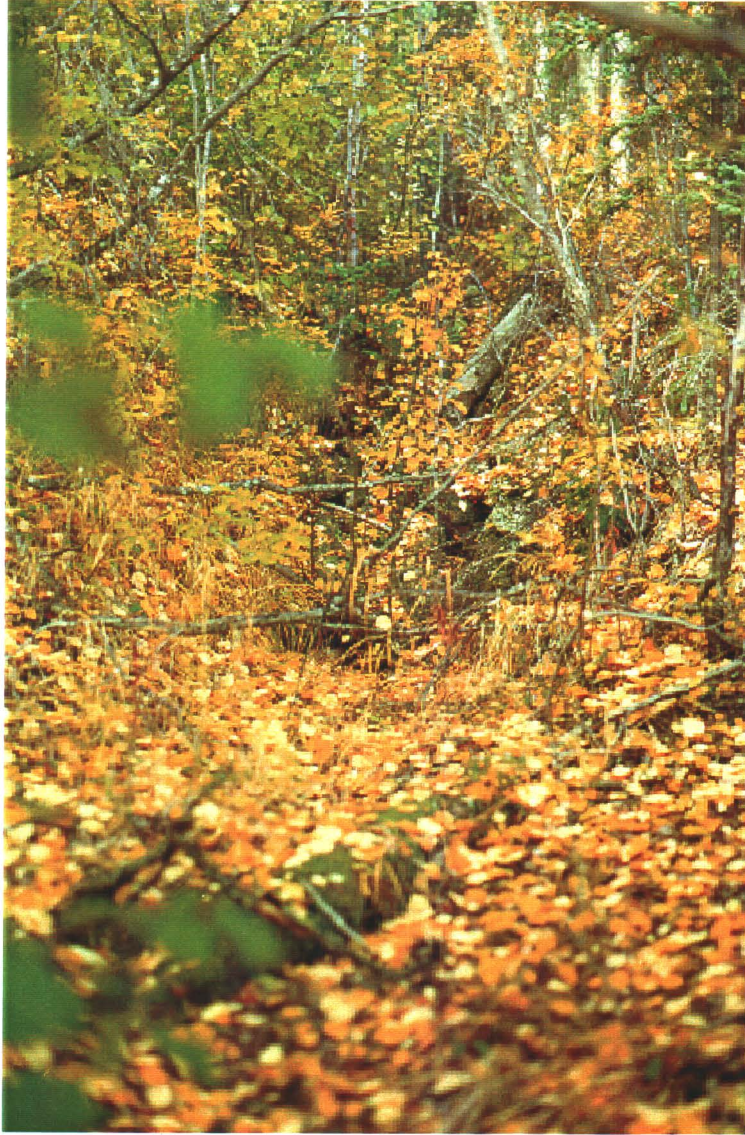
Photo 16-1: Collapsed and overgrown portal and adit are barely visible from under the leaf cover. (Azimuth 270°)
