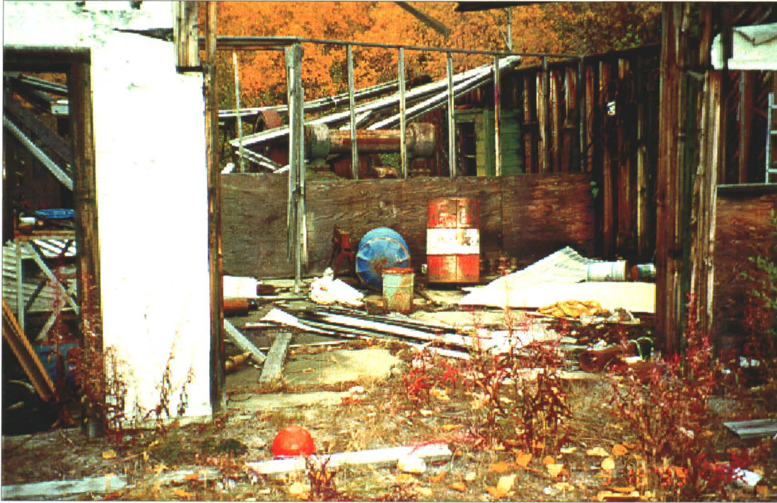
Photo 19-9: Former storage area in building 19E where hazardous liquids stored.
