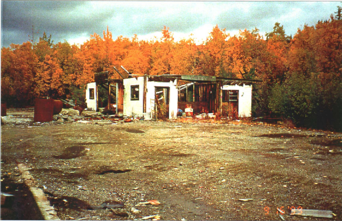
Photo 19-7: Remains of building 19E at lower area. Note oil staining in foreground.
