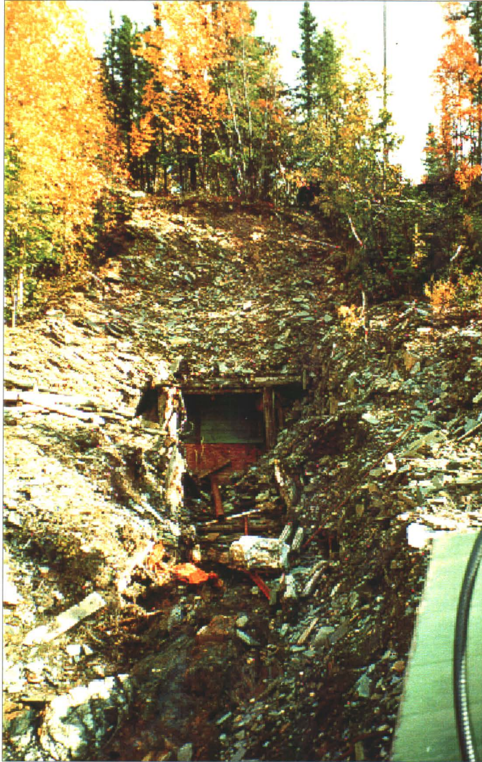
Photo 19-2: 400 level portal and runoff channel. Note debris at entrance.
