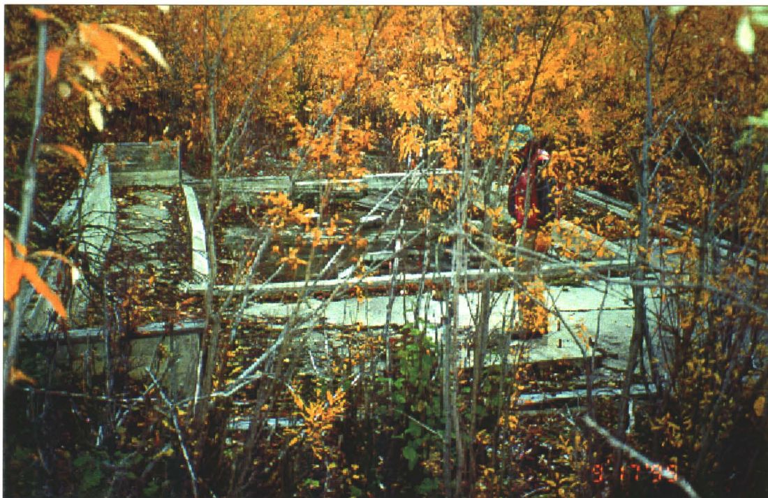
Photo 19-16: Concrete foundation (building 190) at loadout site.
