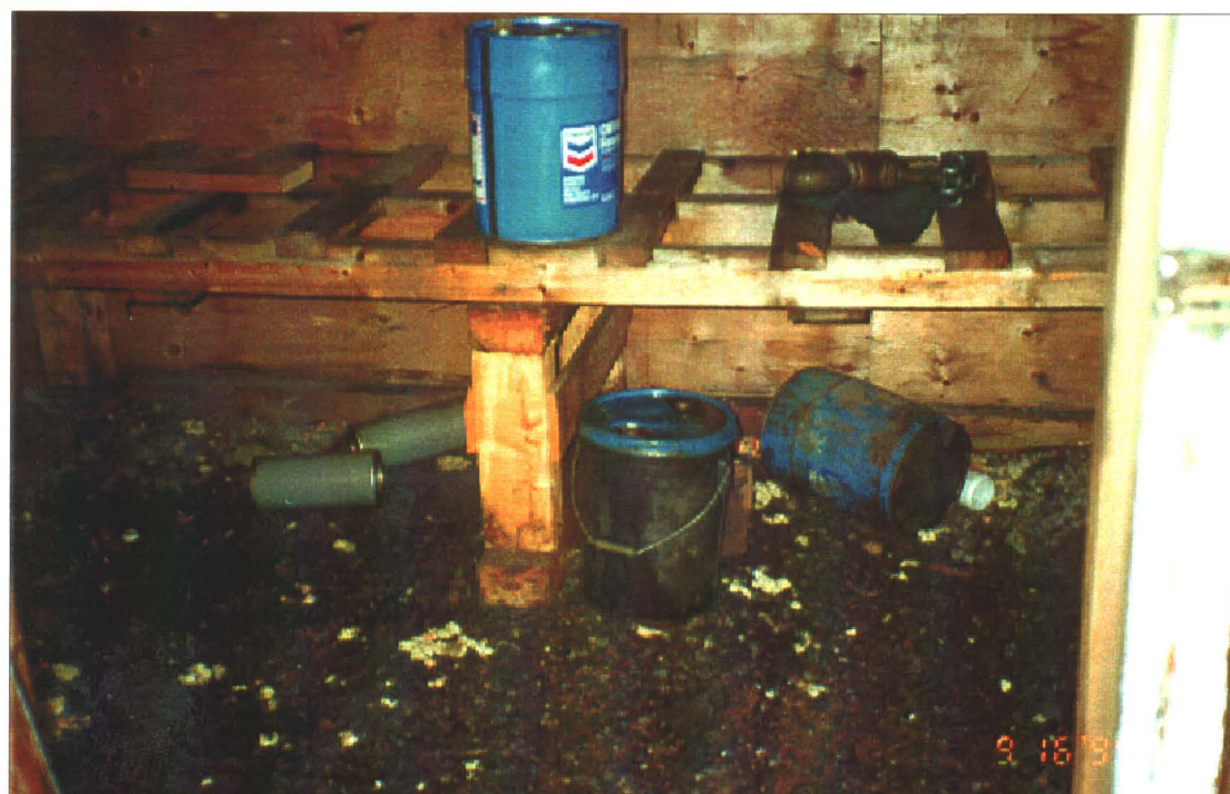
Photo 19-19: Hydrocarbon containers and extensive staining inside building 19C.
