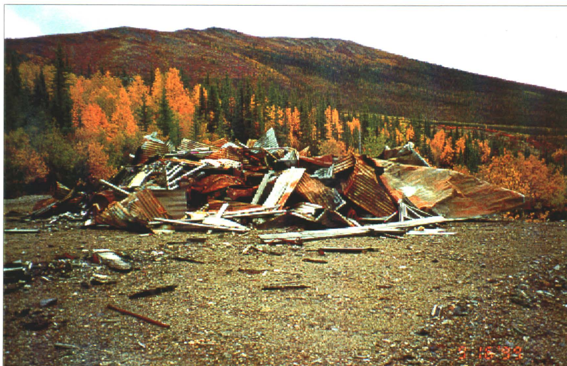
Photo 19-12: Construction waste debris remaining from demolition of building 19G.
