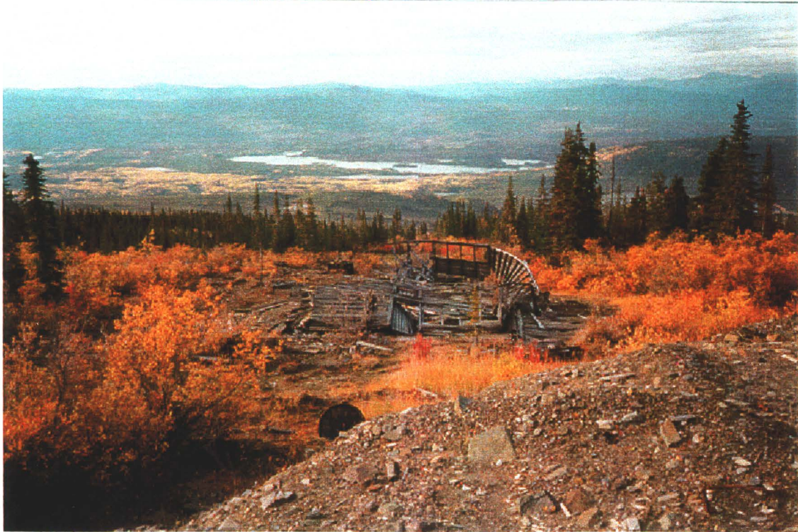
Photo 21-17: Collapsed building (Bldg. 21-J). (Azimuth 320°)
