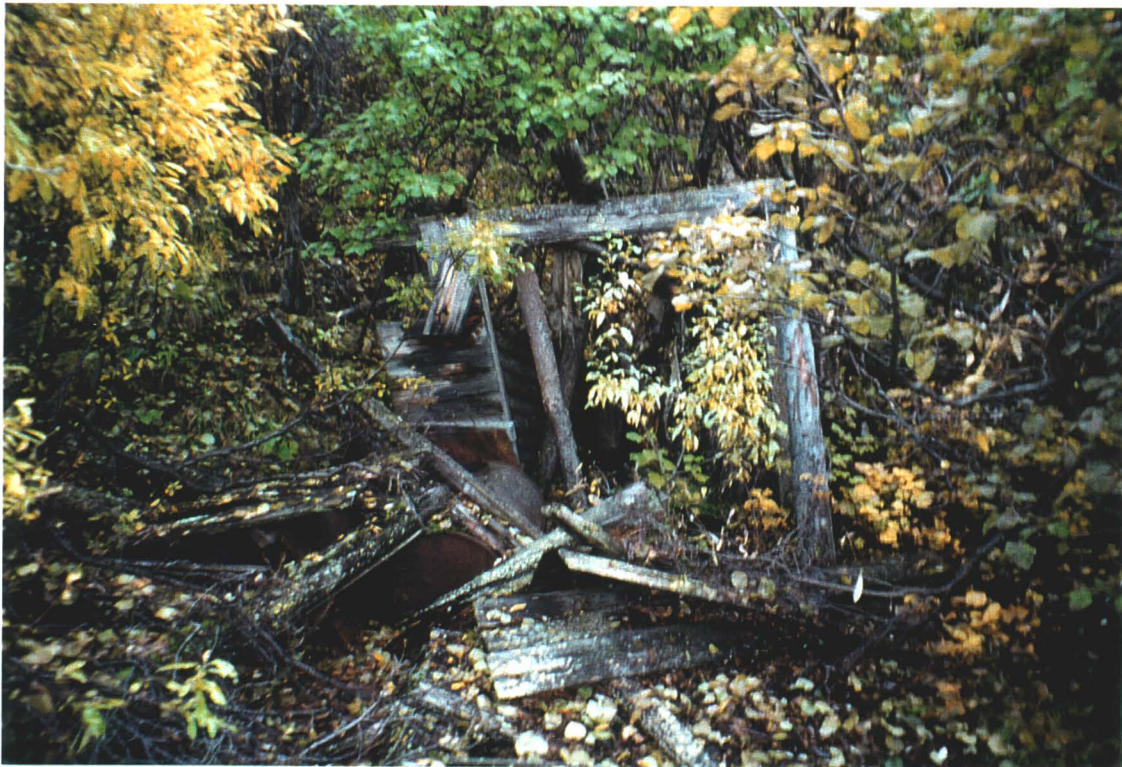
Photo 22-12: View of collapsed entrance to Mayo Mines adit (Azimuth206°)
