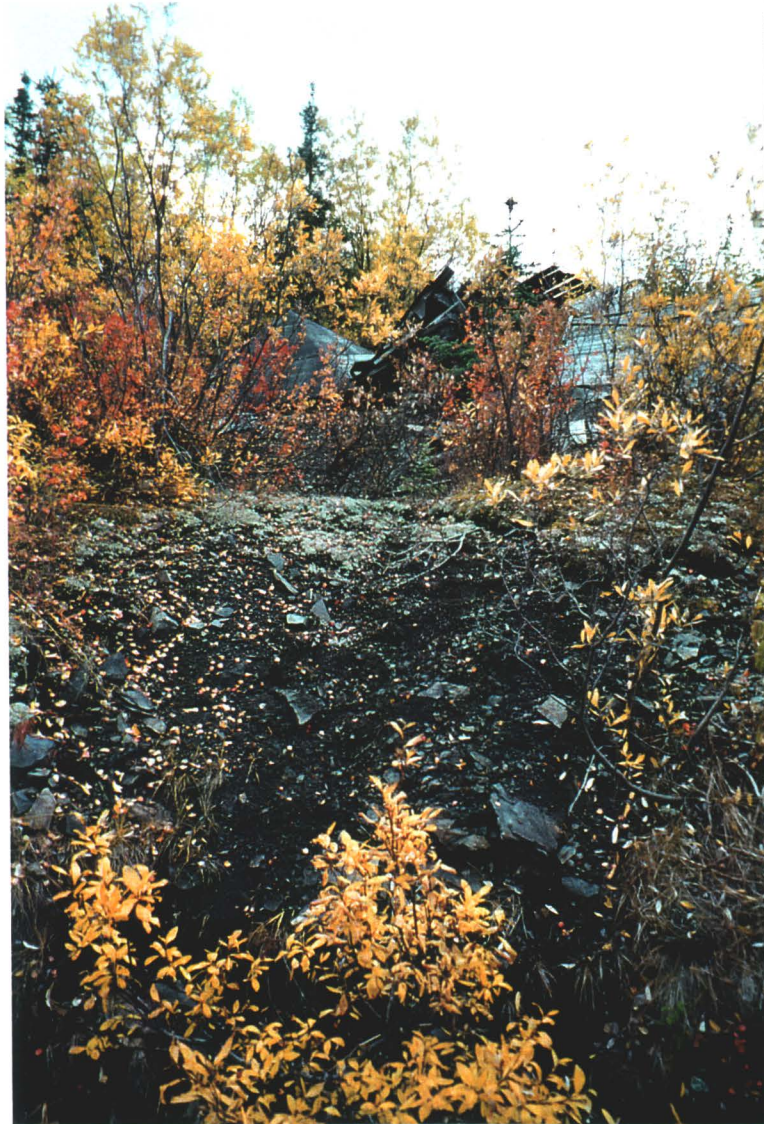
Photo 22-10: Collapsed entrance to Bellekeno 100 level adit with waste rock dump in foreground.
