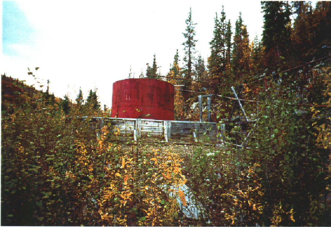
Photo 22-5: Aboveground fuel storage tank behind compressor house at Bellekeno 625 level adit.
