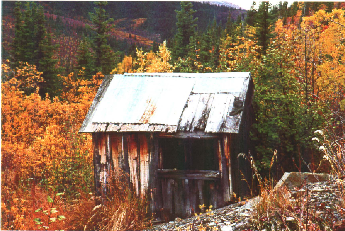
Photo 22-19: Powder shed located adjacent to Eureka Shaft 3.
