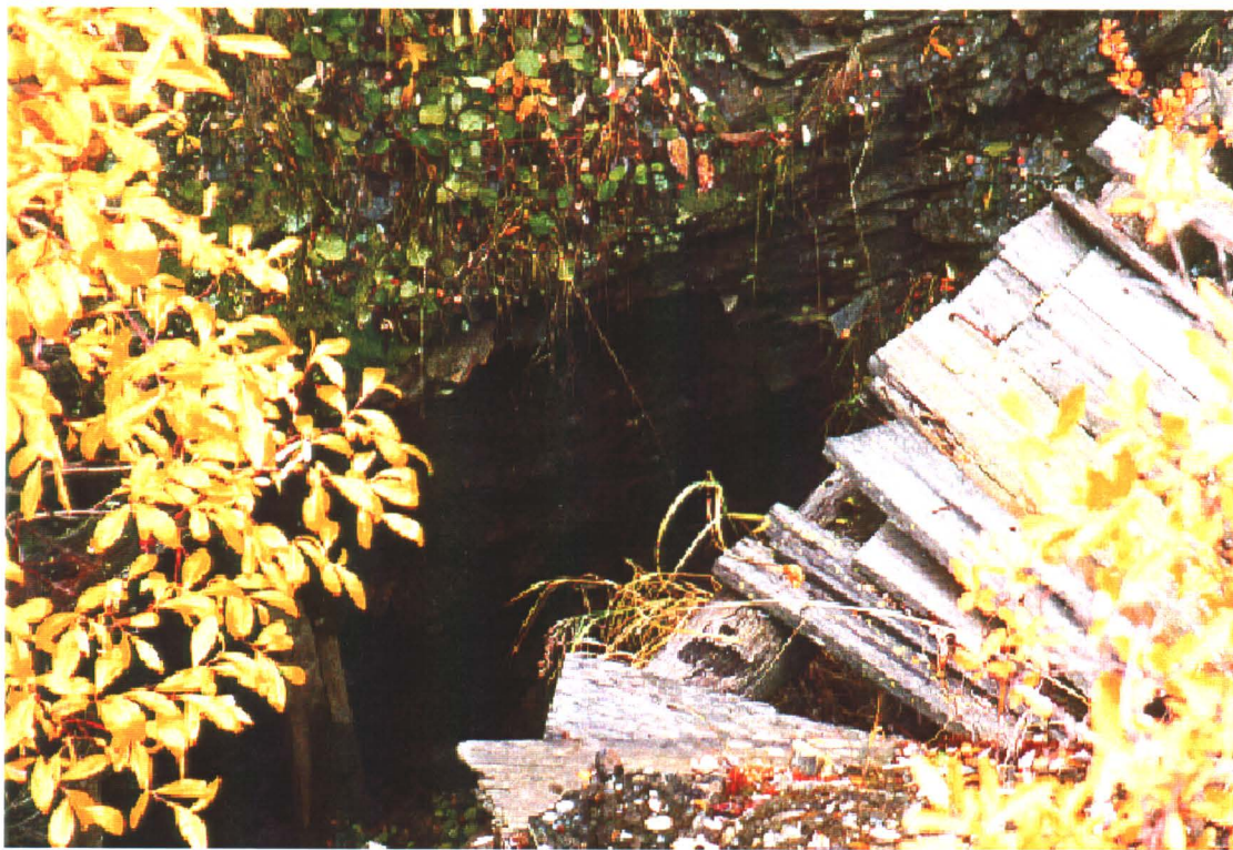
Photo 22-18: Partially collapsed shaft (Eureka Shaft 3) located about 37 m south of Eureka Shaft 1.
