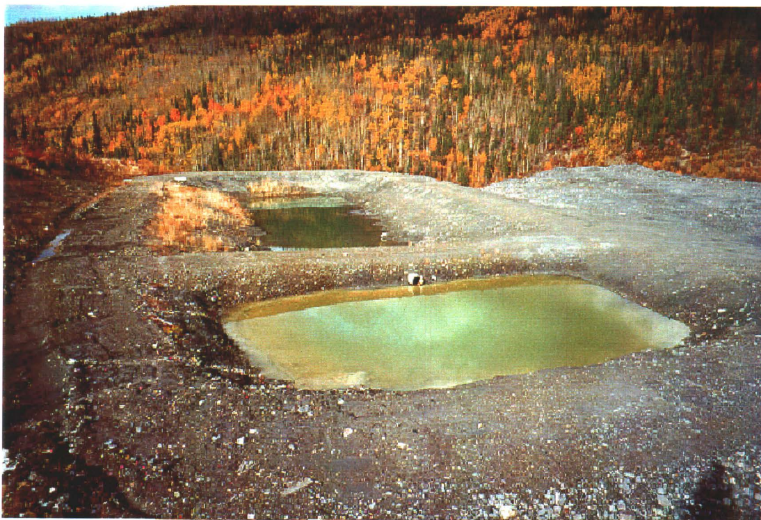
Photo 22-2: Settling ponds for treatment of water removed from Bellekeno mine at 625 level adit.
