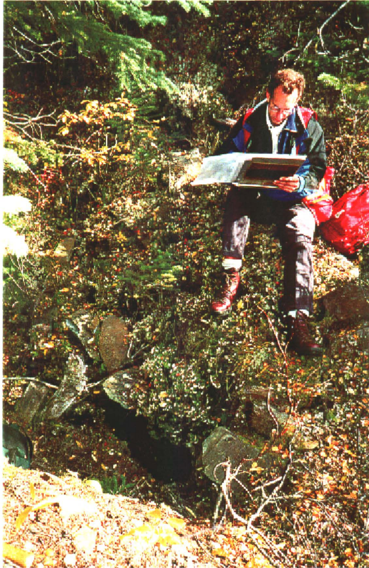
Photo 23-1: Caved lower portal area; note small opening below mapper's feet and natural revegetation of the site. Photo Direction (Azimuth 040°)
