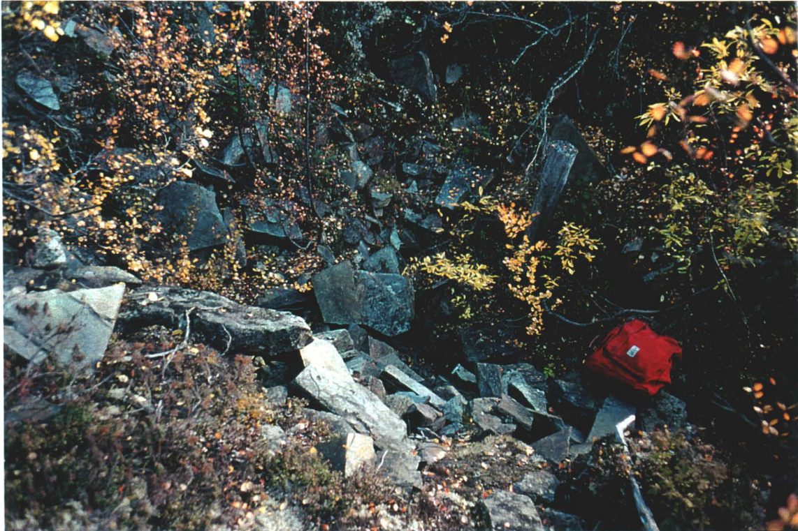
Photo 23-4: Collapsed middle trench and adit area. Note portal timber above pack protruding from angular colluvial greenstone boulders.
