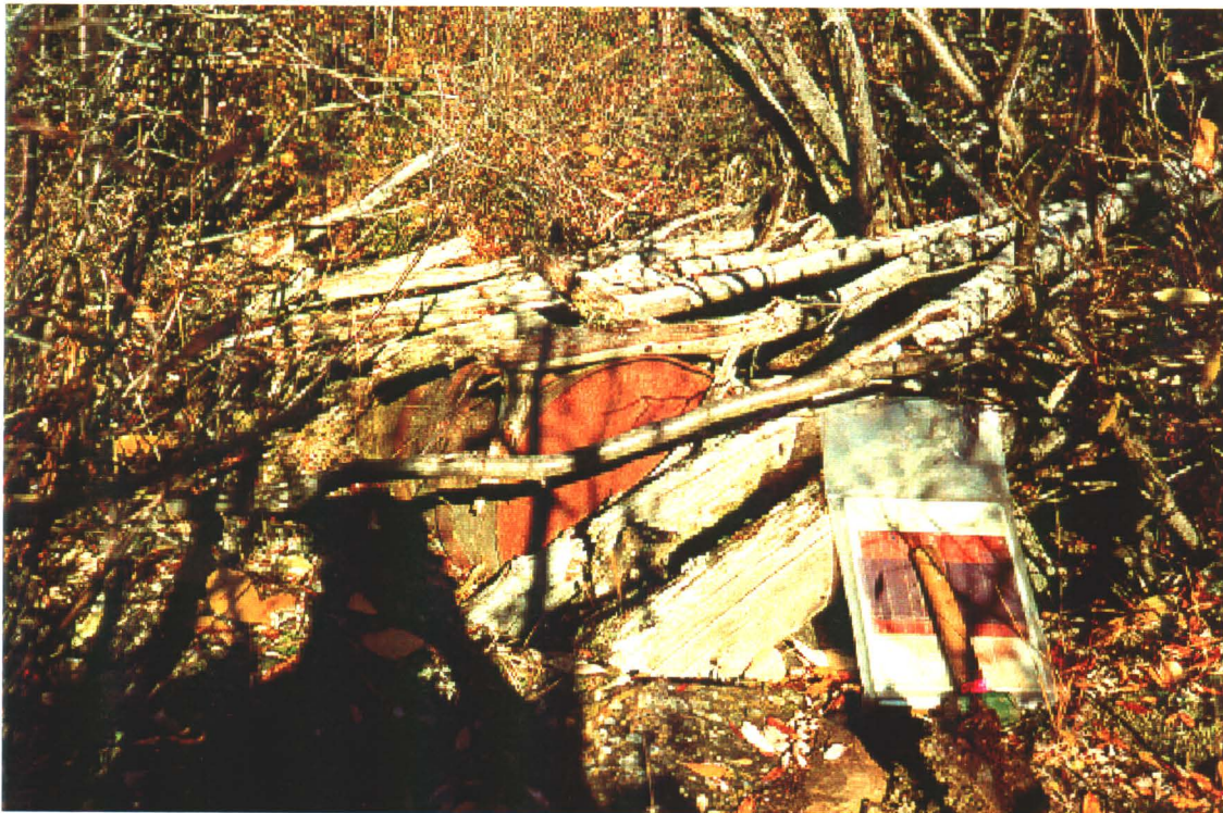
Photo 24-4: Adit #1 portal area. (Azimuth 030°)
