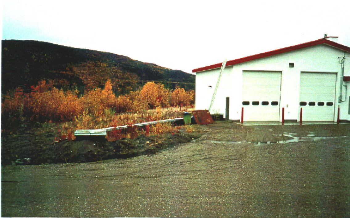
Photo 25-6: Shepherd adit. Note mine drainage dammed behind gravel berm.(Azimuth 090°)
