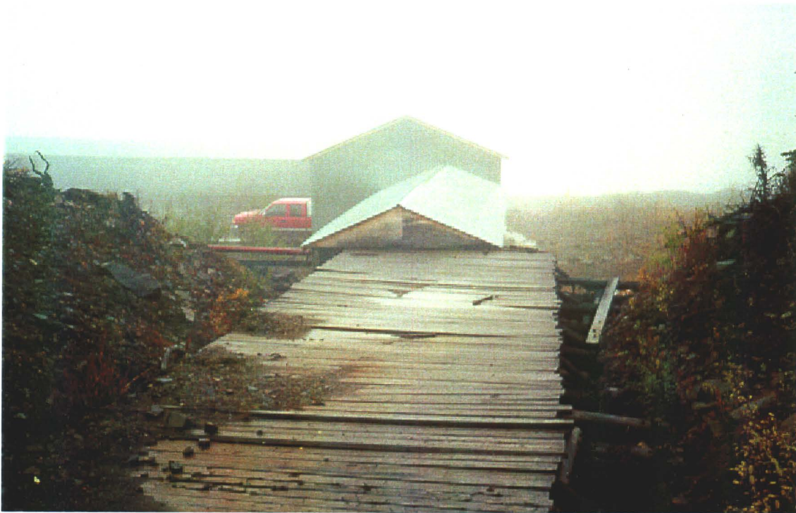
Photo 25-7: Lucky Queen load out building and portal structure. Note cribbed portal in foreground and load-out in background. (Azimuth 200°)
