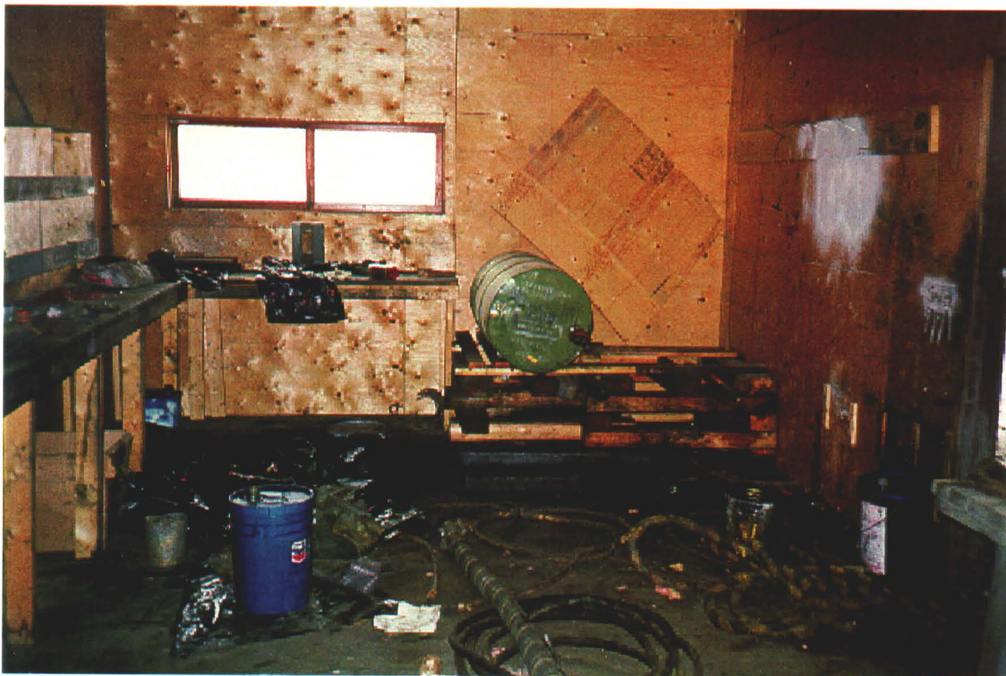
Photo 25-16: Interior of workshop area. Note leaking drum of hydraulic oil and full pan below. (Azimuth 250°)
