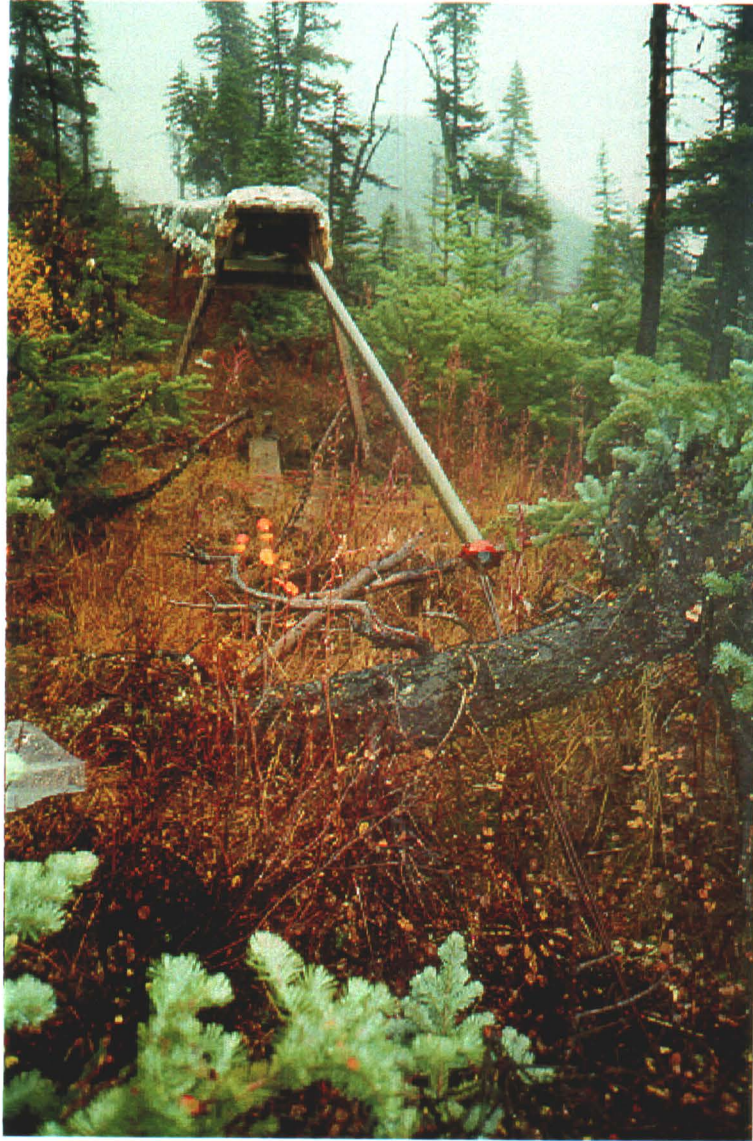
Photo 25-14: Mine drainage flume. Note copper heater coils extending out of pipe. (Azimuth 130°)
