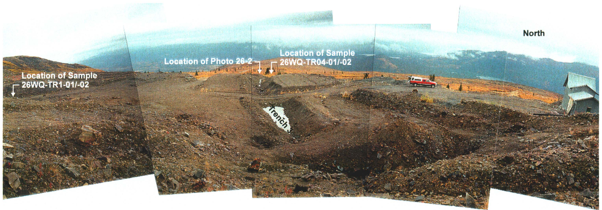
Photo 26-1: Panorama of site showing trenches, shaft building and overburden and waste rock dumps. Note old shaft just left of Trench 3 in foreground and powerline and haulage tram towers in background.
