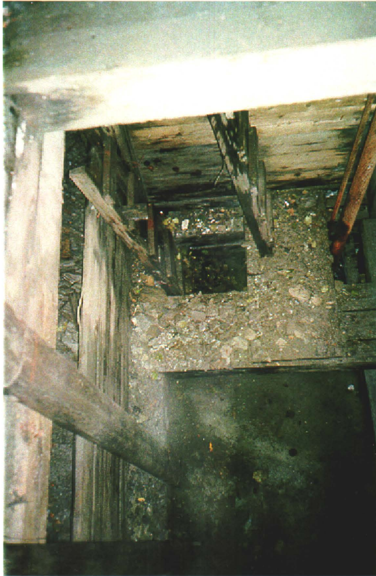
Photo 27-2: Interior of shaft A01 headframe (Bldg. 27-1).
