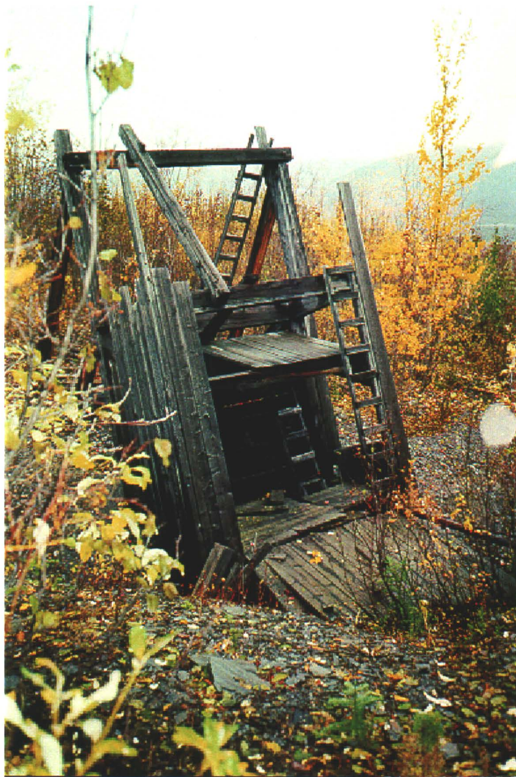
Photo 27-1: Shaft headframe (Bldg. 27-1). (Azimuth 340°)
