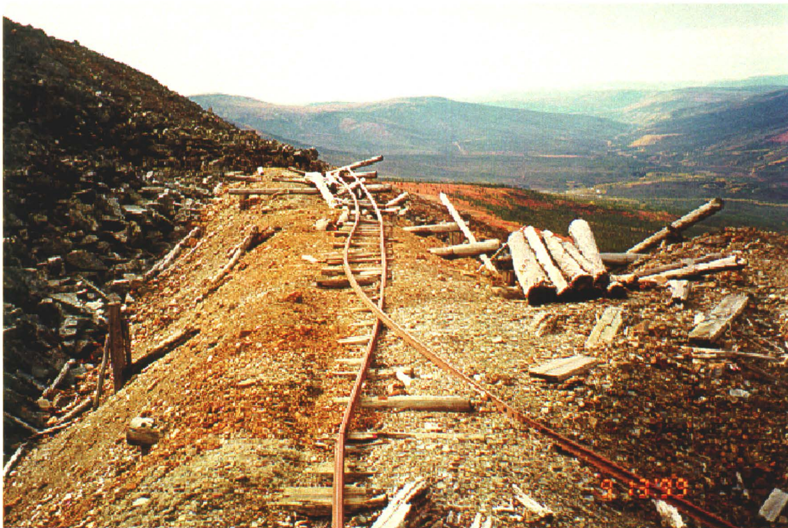
Photo 28-8: Rail and trestle at main adit.
