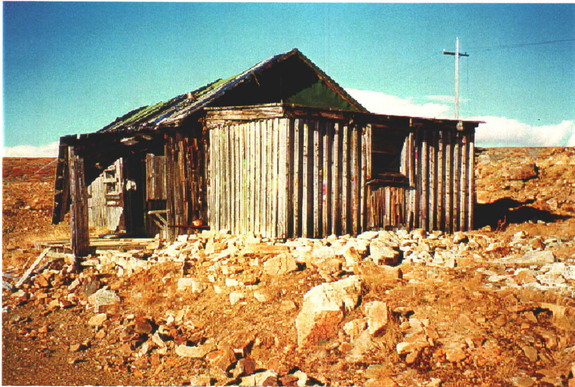
Photo 28-5: Main site living quarters (building 28A).
