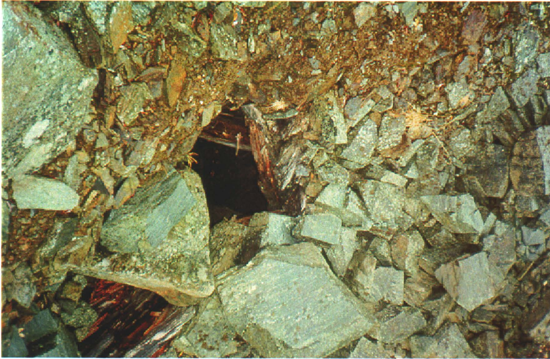
Photo 29-2: Northern partly collapsed adit, upper workings.
