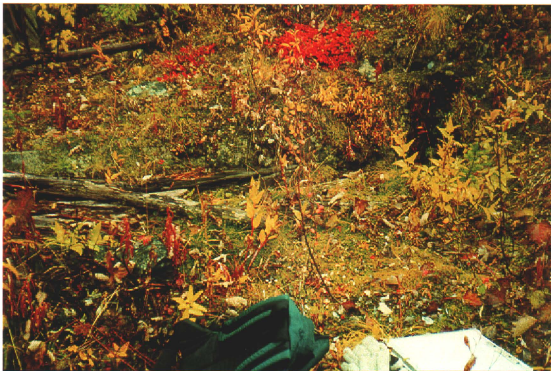
Photo 29-5: Collapsed adit, lower workings."
