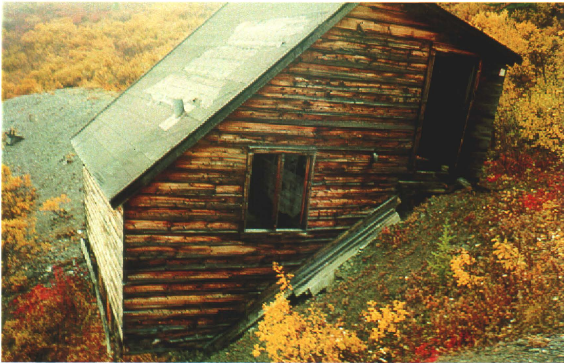
Photo 29-7: Ore processing building.
