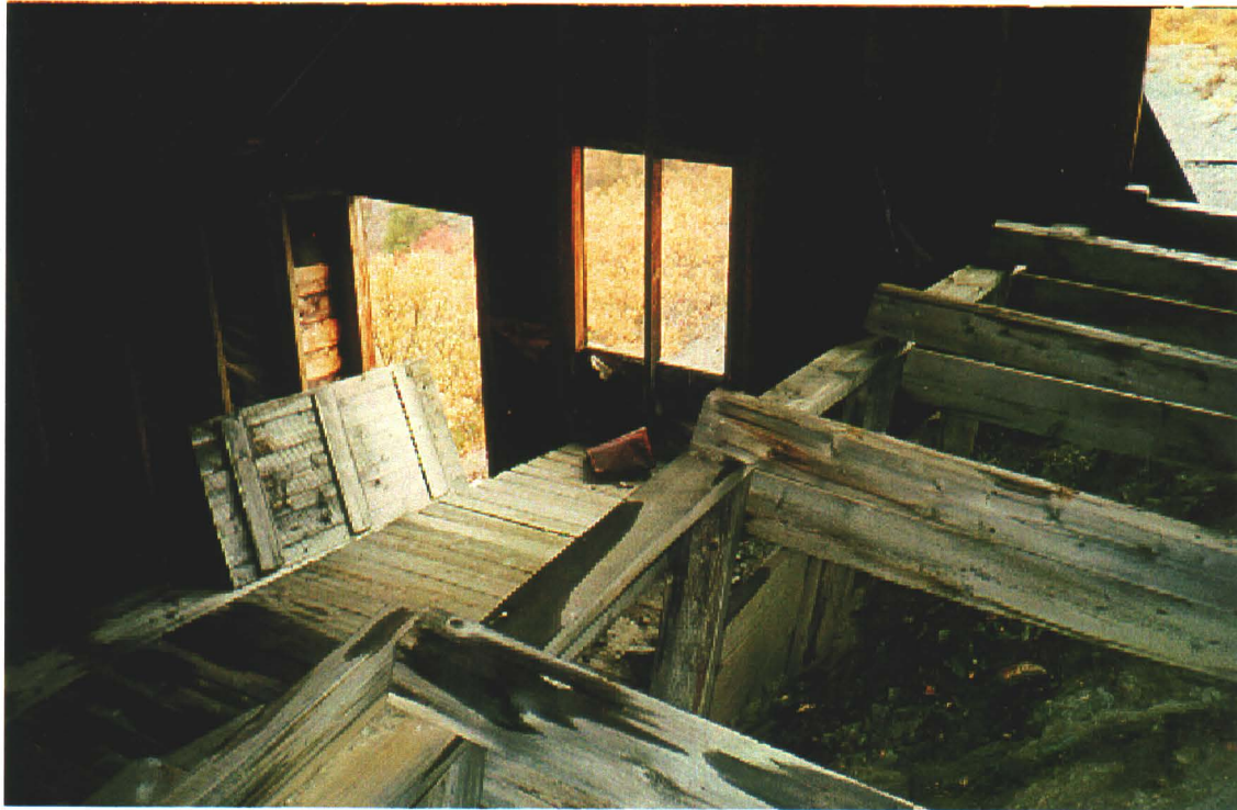
Photo 29-9: Interior of ore processing building.
