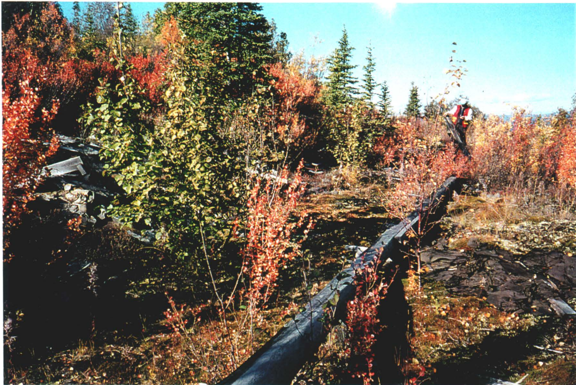
Photo 31-8: Demolished buildings (Bldgs. 31-C, D) along road west of Stone. Note discarded asbestos containing siding at right and in background held by field personnel. at depth in pit and abundant siderite vein cobbles. Photo Direction (Azimuth 290°)
