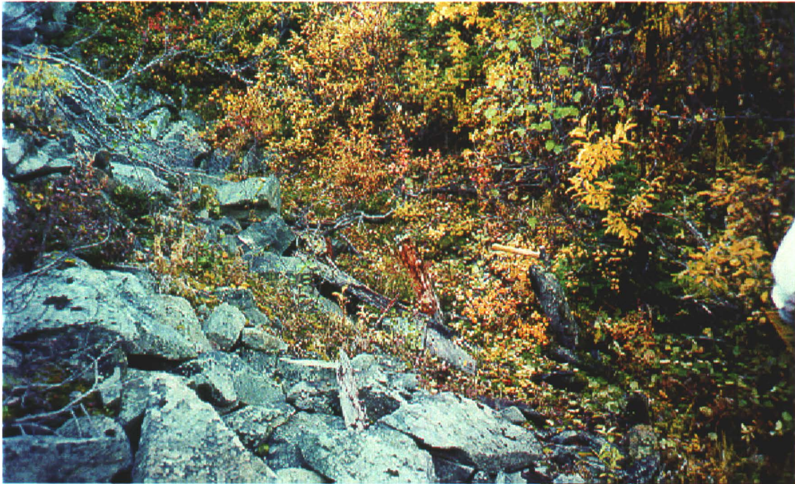
Photo 31-2: Collapsed upper adit portal. Note hammer in old portal timbers. Photo Direction (Azimuth 230 o )
