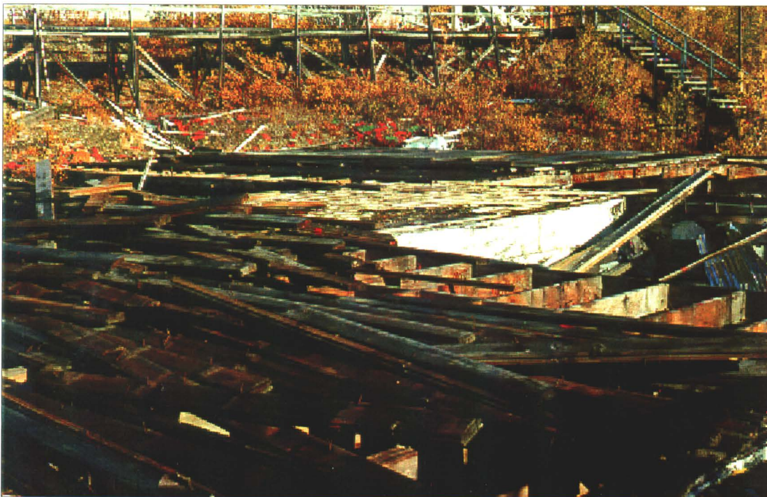
Photo 32-14 : Keno 700. Old bunkhouse site (building 3) looking north.
