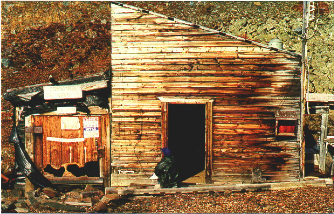
Photo 32-5 : Comstock-Keno 150. Adit Shack (looking N.).
