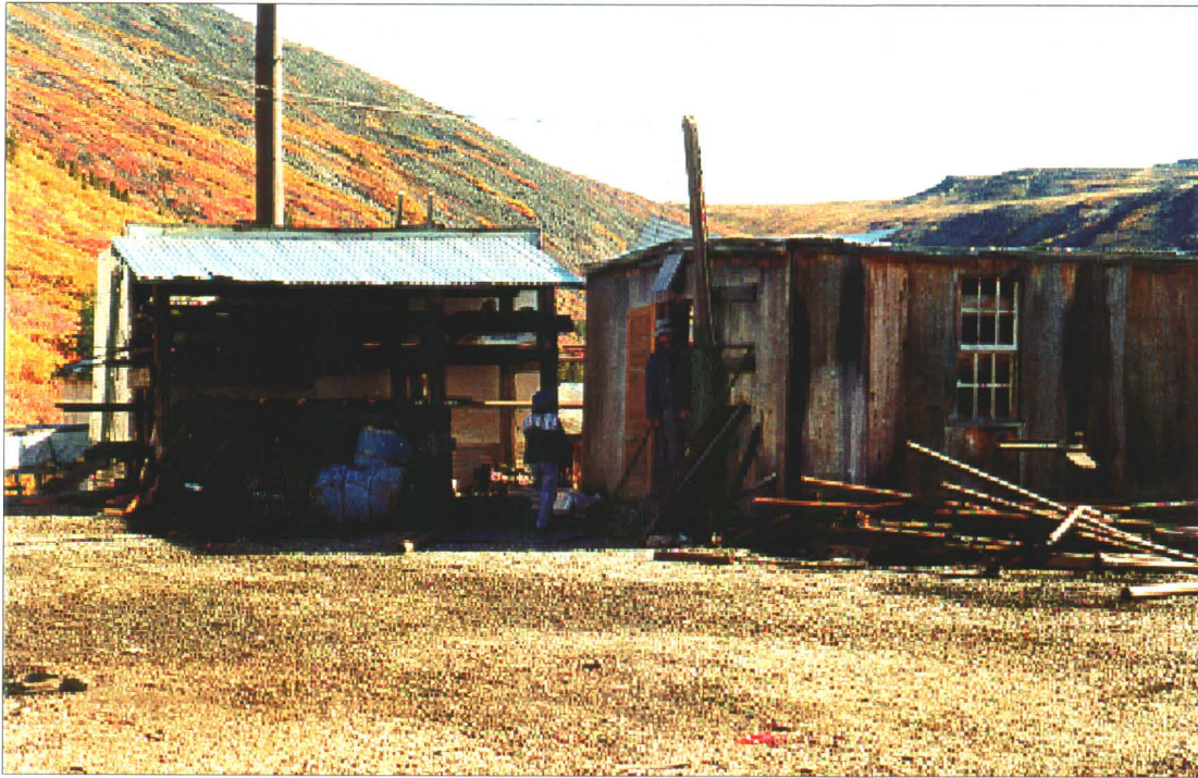
Photo 32-19 : Keno 700. Paint shed (building 10) looking E.
