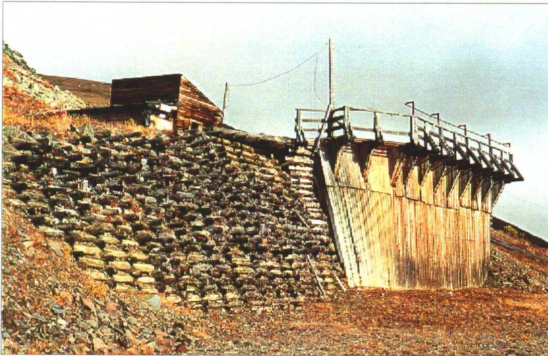
Photo 32-23 : Comstock-Keno 150. Adit shack & truck-loading trestle.
