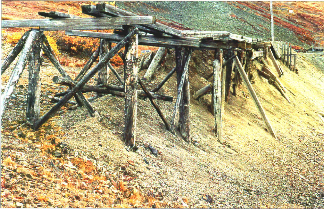
Photo 32-11 : Keno 200. Old trestle to S.W. of site looking N.E.
