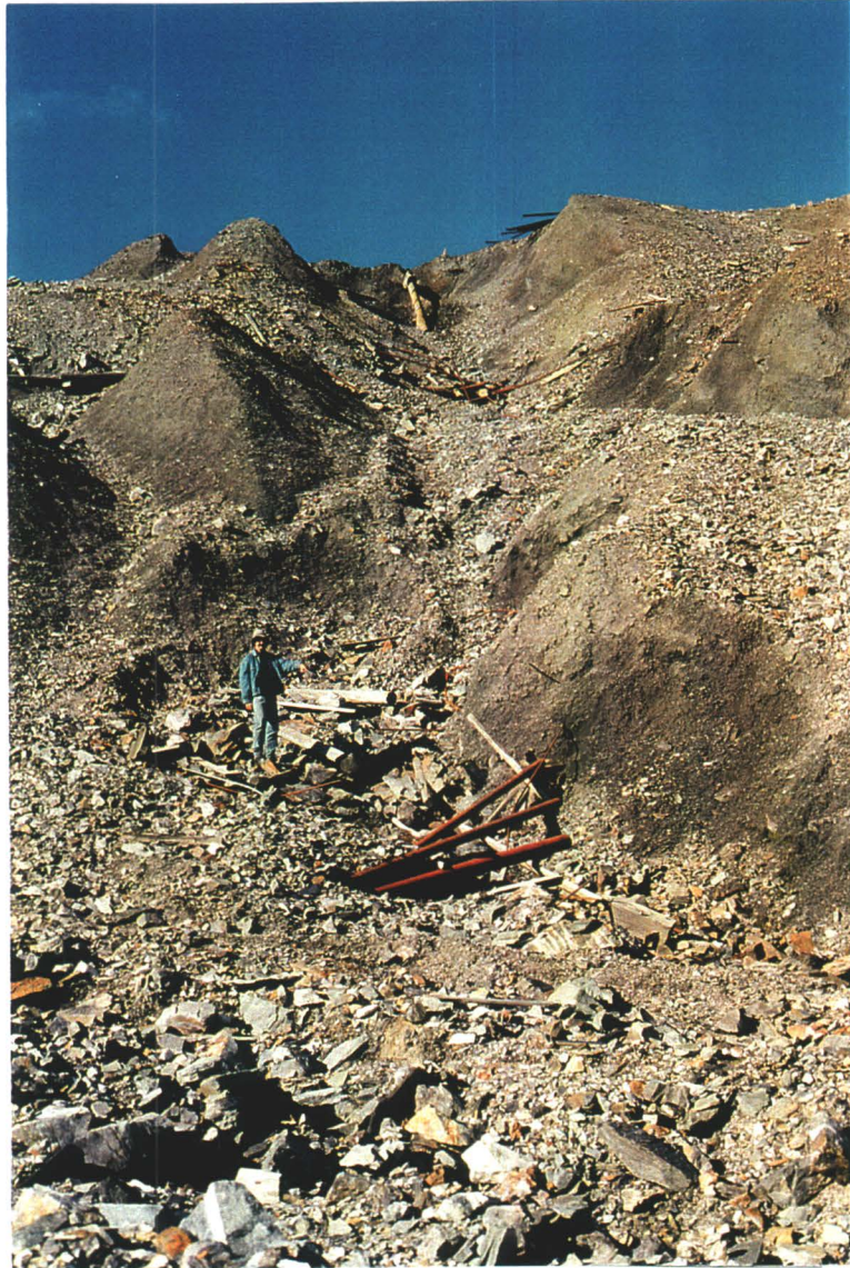
Photo 32-28 : Keno 700. Waste-rock pile outwash area looking W. Adit culvert at top.
