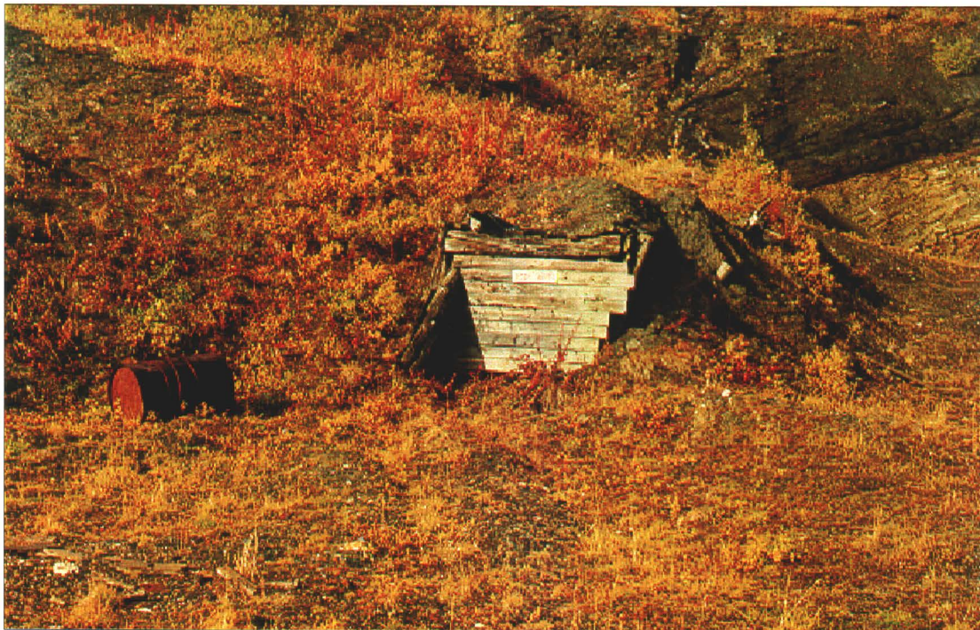
Photo 32-8 : Porcupine Adit looking N.W.
