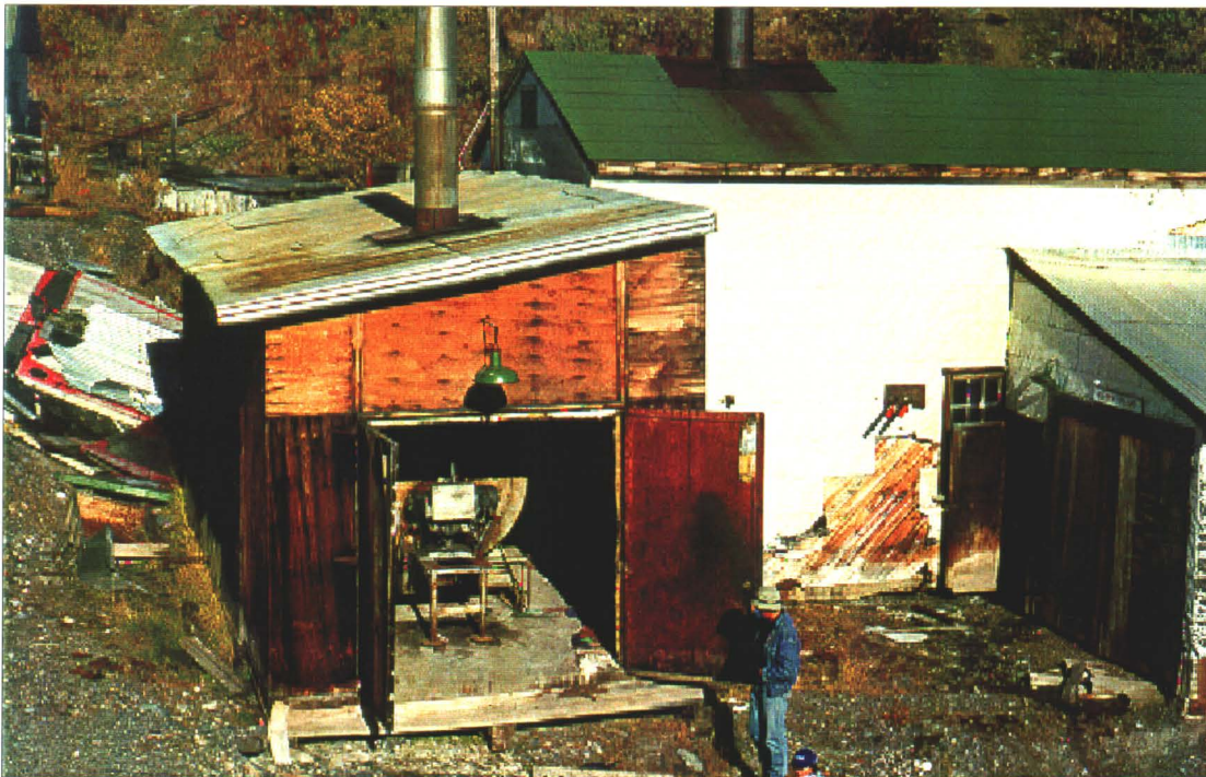
Photo 32-20 : Keno 700. Boiler shack / filter plant (building 12) looking N.E.
