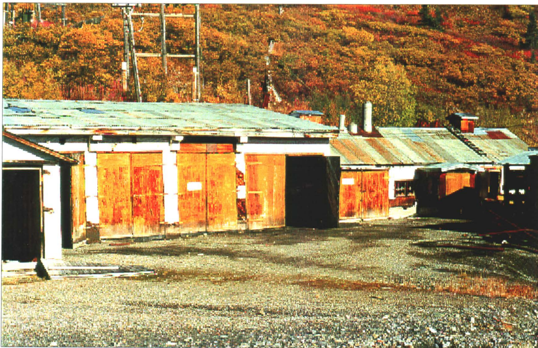
Photo 32-18 : Keno 700. Generator shack (building 9) looking north - oil staining in front.
