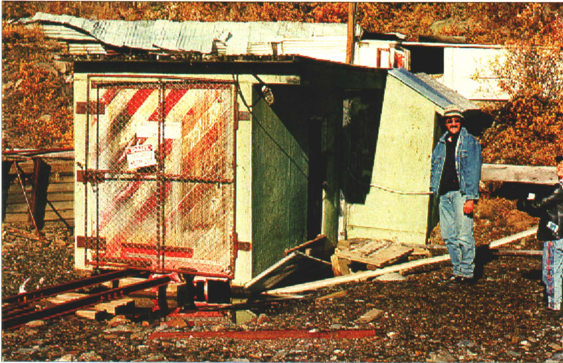
Photo 32-2 : Keno 700. Mine adit shed (building 7) looking N.W.
