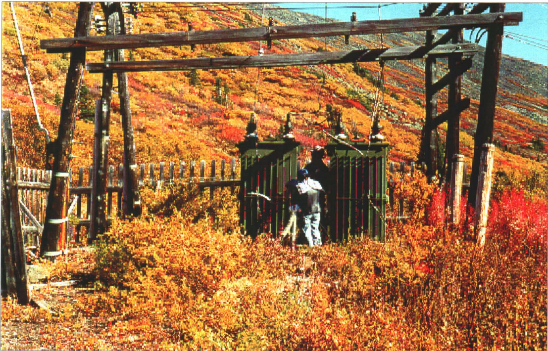
Photo 32-25 : Keno 700. Transformer site looking N.E.
