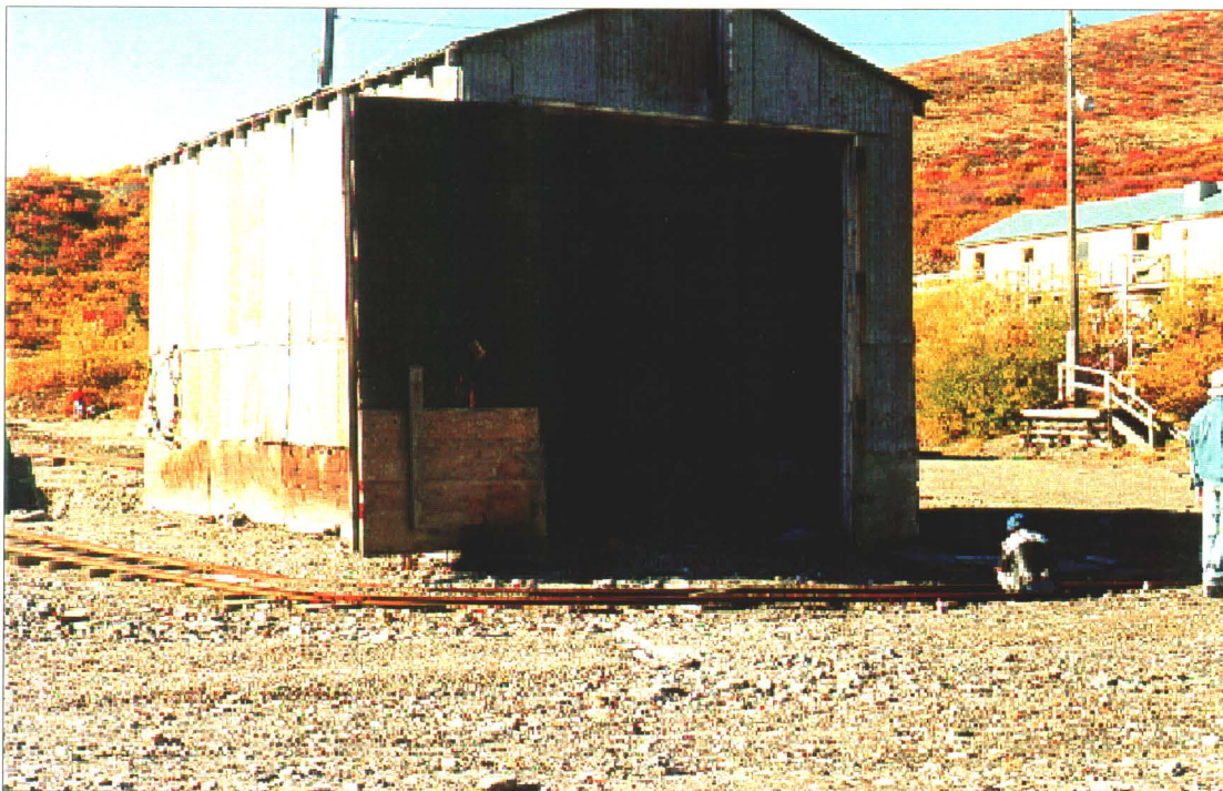
Photo 32-16 : Keno 700. Vehicle maintenance shed (building 6) looking S.W.
