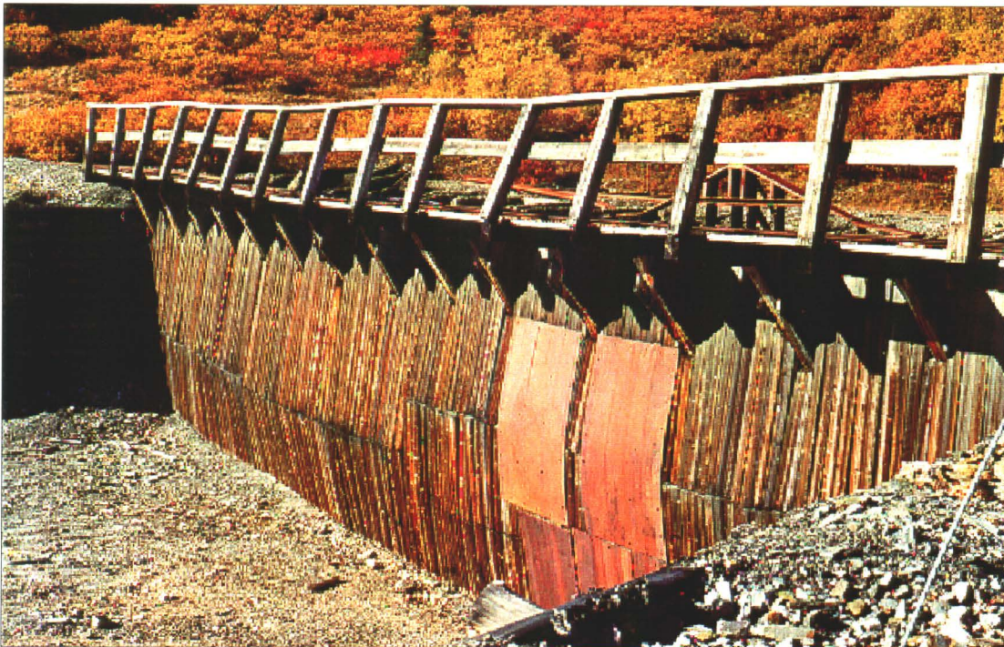
Photo 32-22 : Keno 700. Truck loading trestle at S. end of site.
