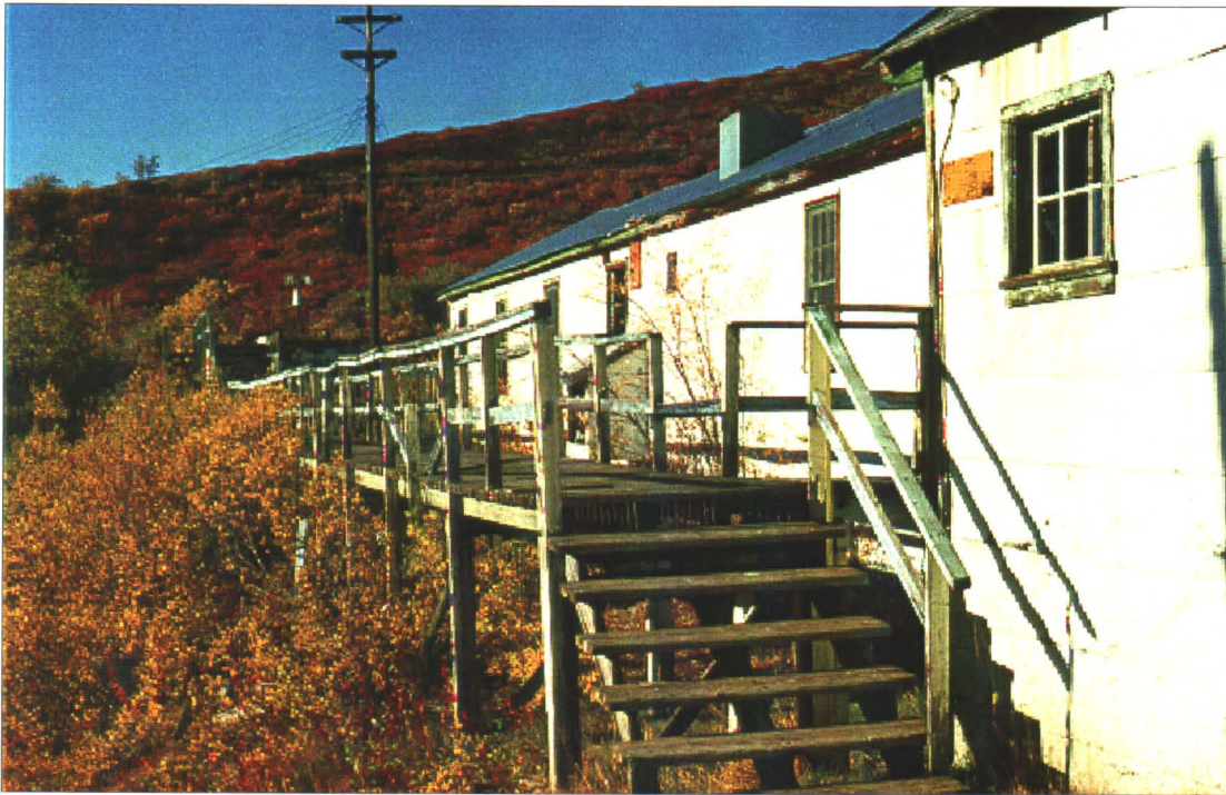
Photo 32-13 : Keno 700. Mess hall facing south (building 2).
