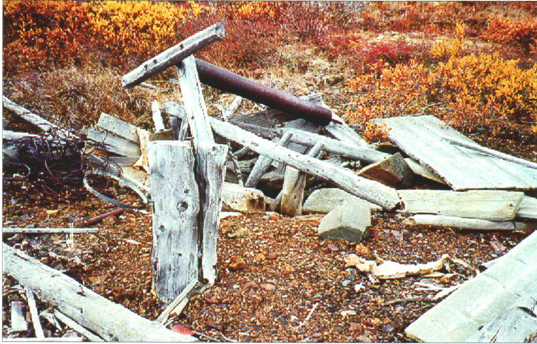
Photo 35-1 : Nabob #2. View of the collapsed Nabob #2 shaft. (Azimuth 050°)
