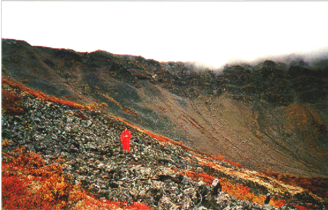
Photo 36-4 : Keno No.9 Faro Gulch cirque headwall with Faro Gulch Portal / Dump shed visible above person. Cuts along skyline left of person are (from left to right), No. 9 Vein and No.3 Vein Pits. Note waste rock dumps associated with each of the Pits and the Portal. Also note meltwater channels in waste rock from the No.3 and No.9 Vein Pits.
