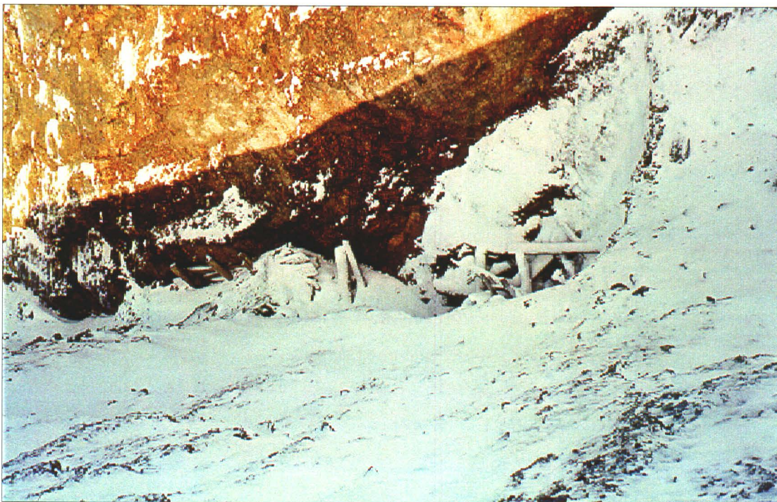
Photo 36-3 : Keno No.9 The log square sets and ladders of the No.3 Vein Adit exposed in the bottom of the No.3 Vein Pit. (Azimuth ~350° )
