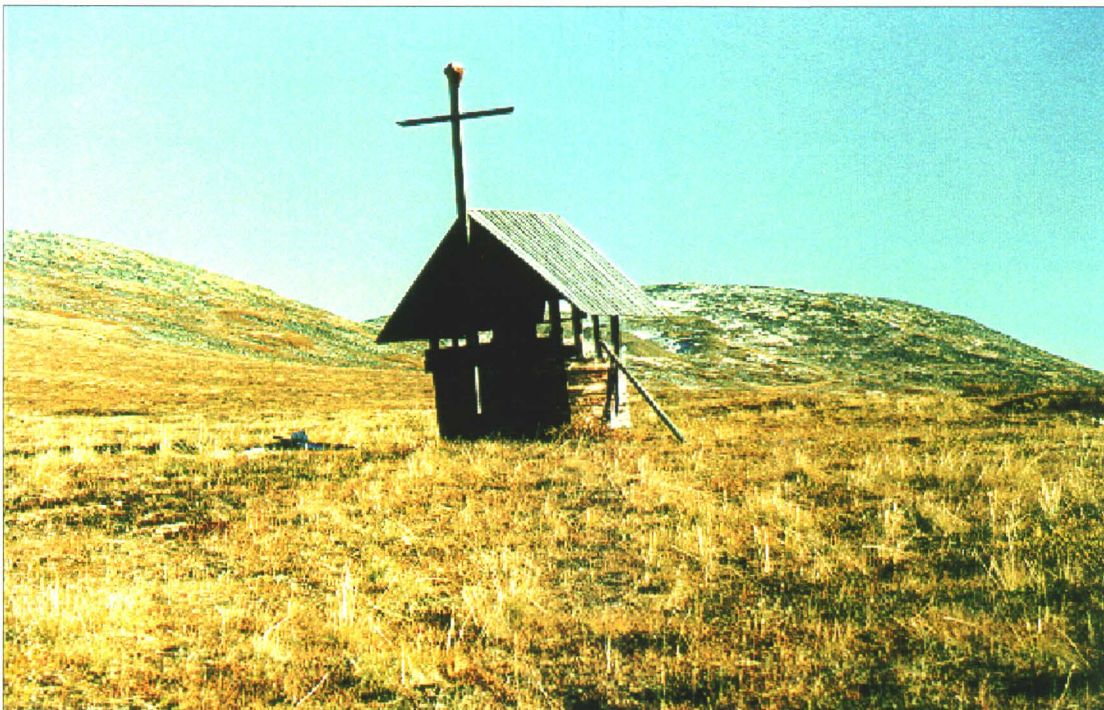
Photo 40-4 : Divide. View of Building 40A. (Azimuth ~050 °)
