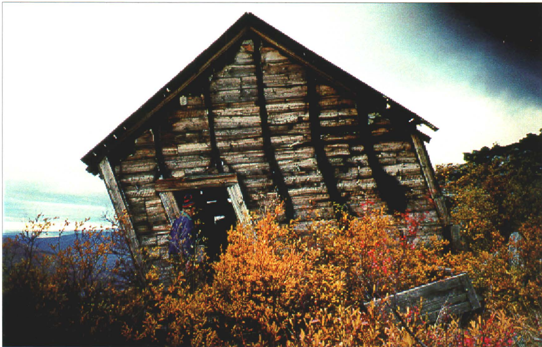
Photo 41-2 : Devon. Building 41A, located 10m south of the Adit.. (Azimuth 280°)
