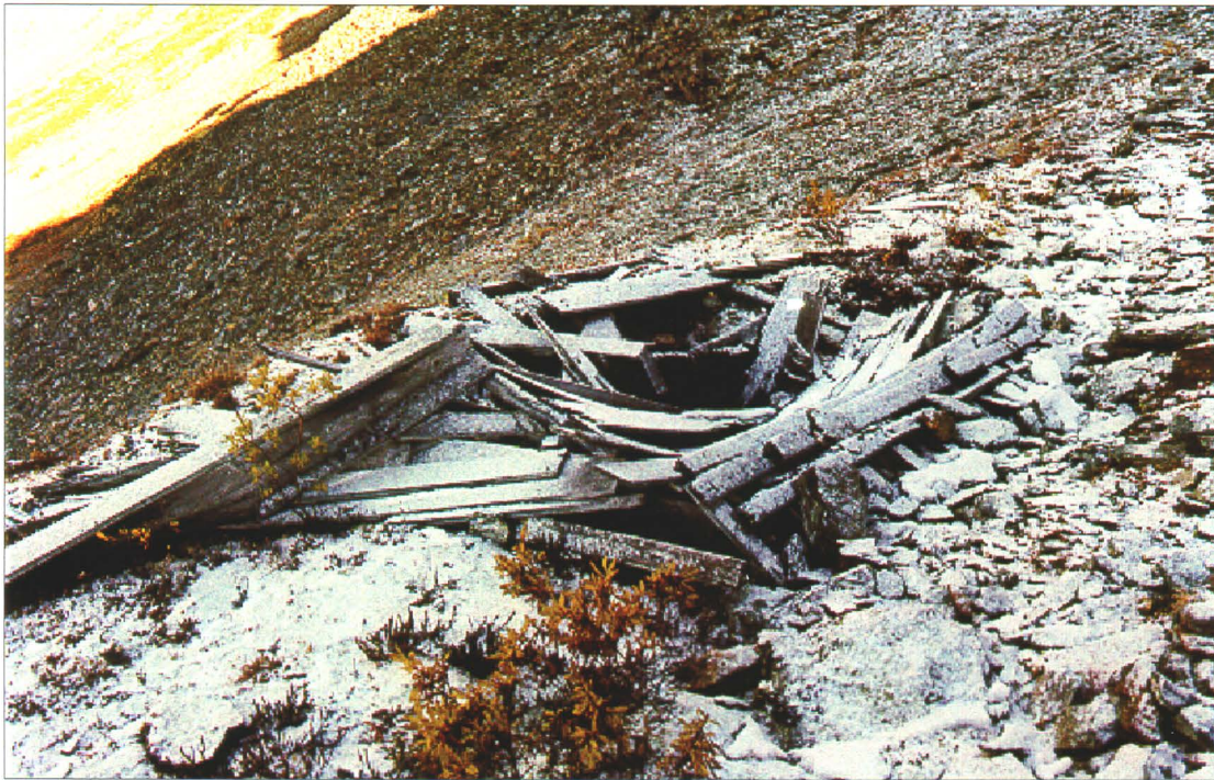
Photo 43-1 : Duncan. Collapsed shaft with windlass still in place across the top. (Azimuth \sim 090^\circ )
