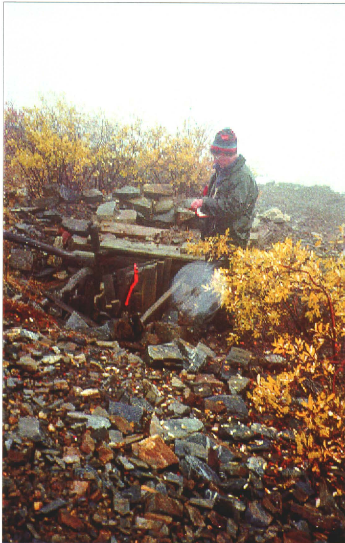
Photo 49-2 : Vanguard. The log cribbing supporting the collar of Shaft #3 is still in place but the shaft has caved 2m below surface. (Azimuth 180 o )
