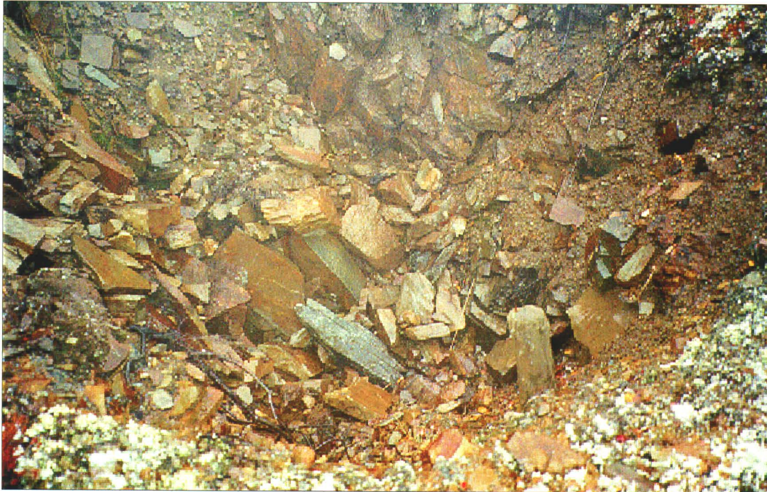
Photo 49-1 : Vanguard. Shaft #2 has collapsed 1m below surface, the timber post in the bottom right hand corner is all that marks the location. (Azimuth 110 o )
