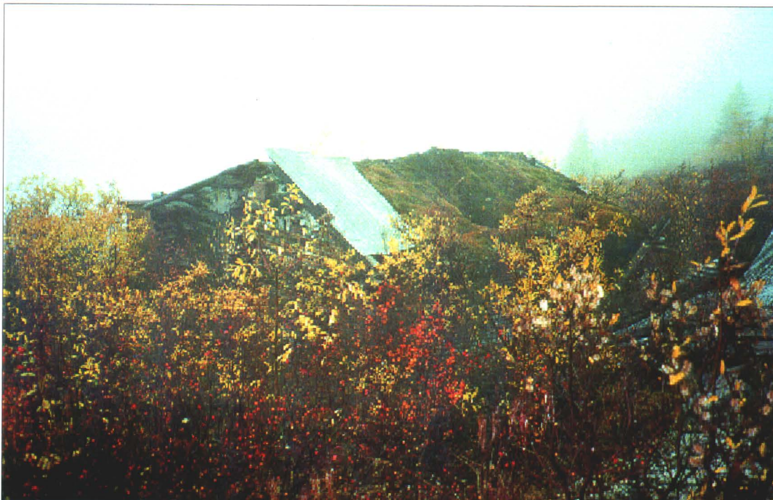
Photo 49-8 : Vanguard. Some rail is still in place but most of it is piled off to the sided. (Azimuth 135 o )
