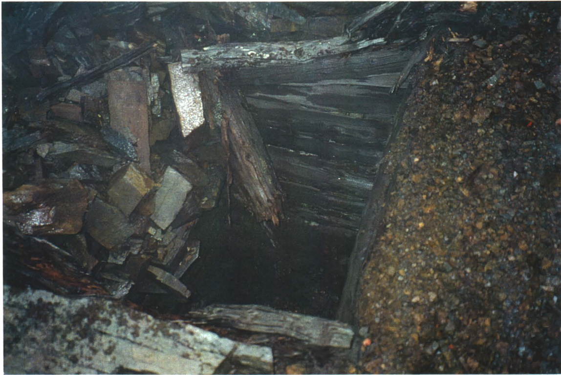
Photo 49-3 : Vanguard. Shaft #4 is still open and in fairly good condition.
