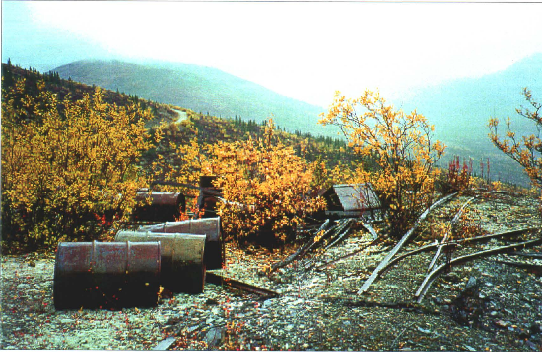
Photo 49-7 : Vanguard. View of Building 49A. (Azimuth 250 o )
