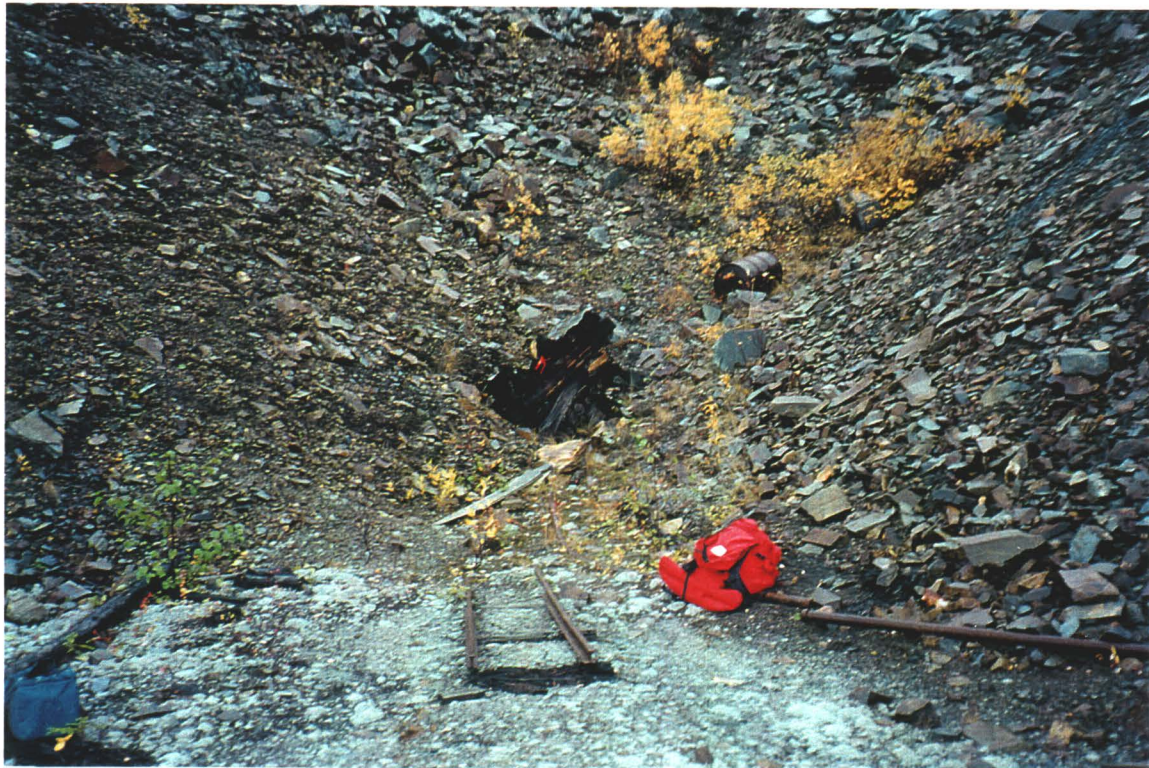
Photo 49-4 : Vanguard. The pile of broken logs and sheet metal marks the entrance to the Vanguard Adit. The first 30m of the adit have collapsed. (Azimuth 290 o )
