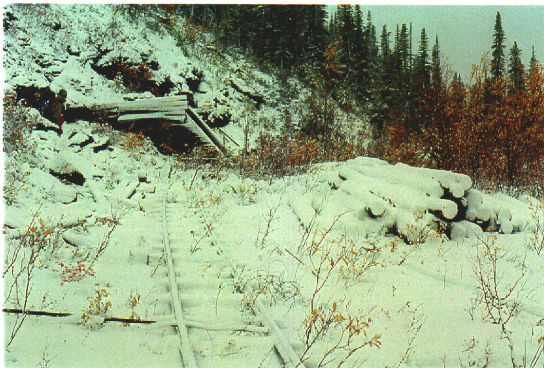
Photo 50-8: Rail and ties, old poles on right and portal to adit in the background. (Azimuth 270°)
