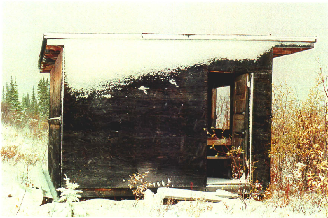
Photo 50-7: Building 50B, the table is visible through the doorway. (Azimuth 270°)
