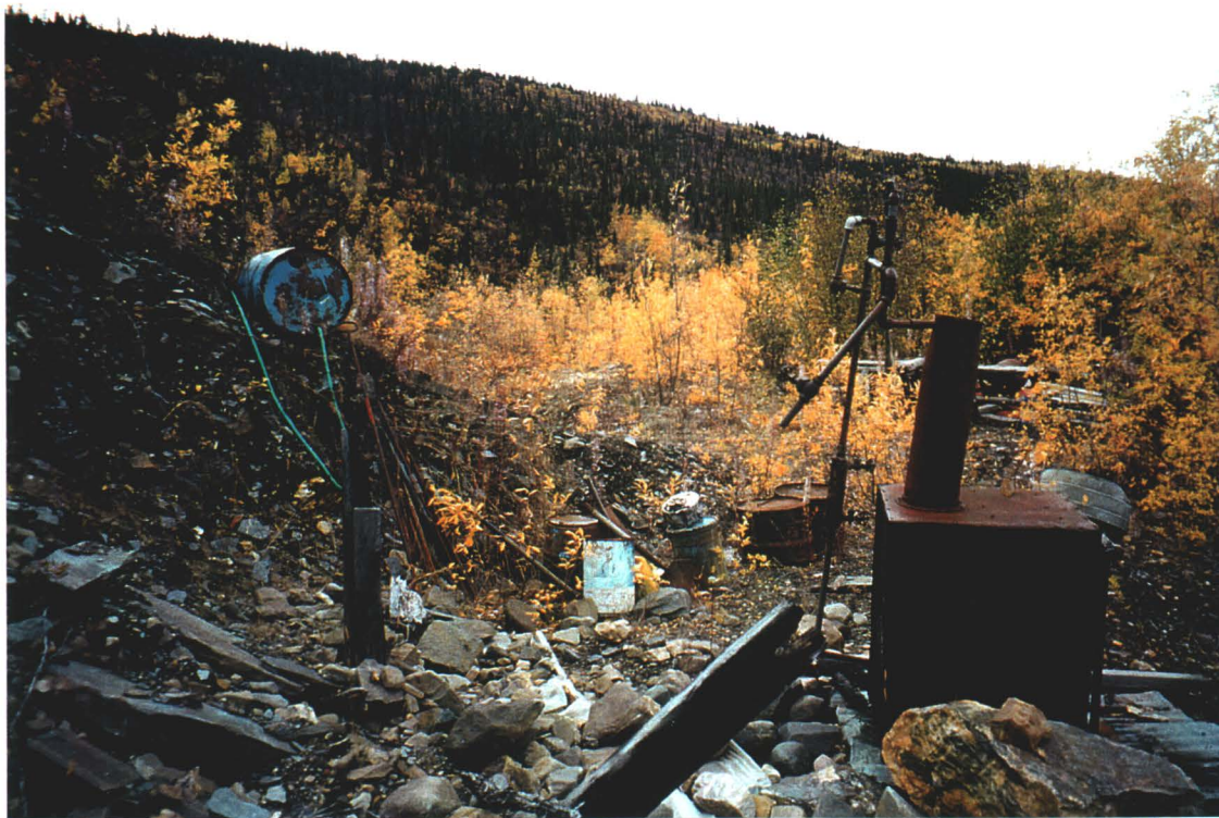
Photo 53-2: View of Adit 1 at Maybrun site. AZ 234 Photo 53-2:View of collapsed shaft (Shaft 1) at Maybrun located above Adit 1.(AZ 300)
