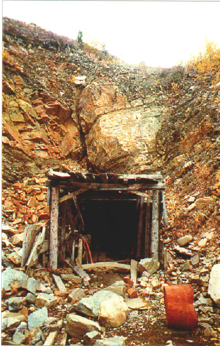
Photo 53-1: View of Adit 1 at Maybrun site. ( AZ 234)
