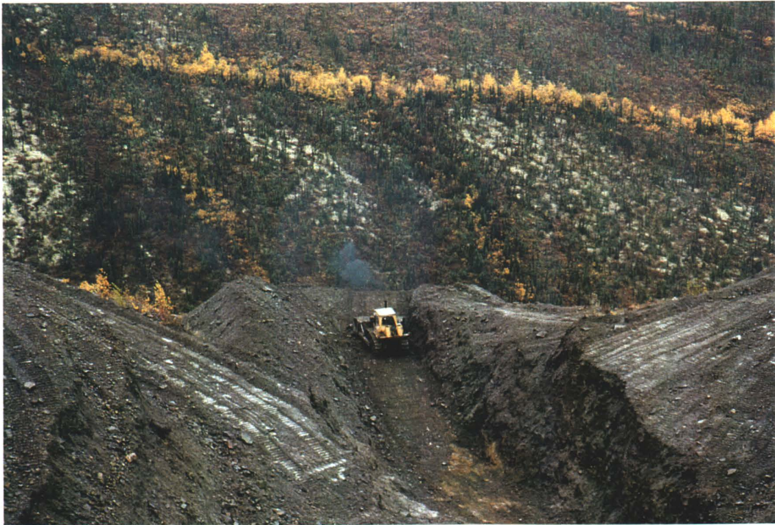
Photo 55-1: Bulldozer working at Runer site.
