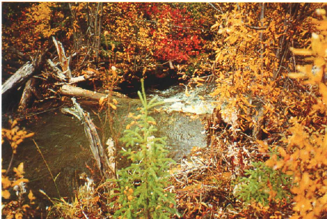
Photo 58-9: Second collapsed bridge downstream of site.
