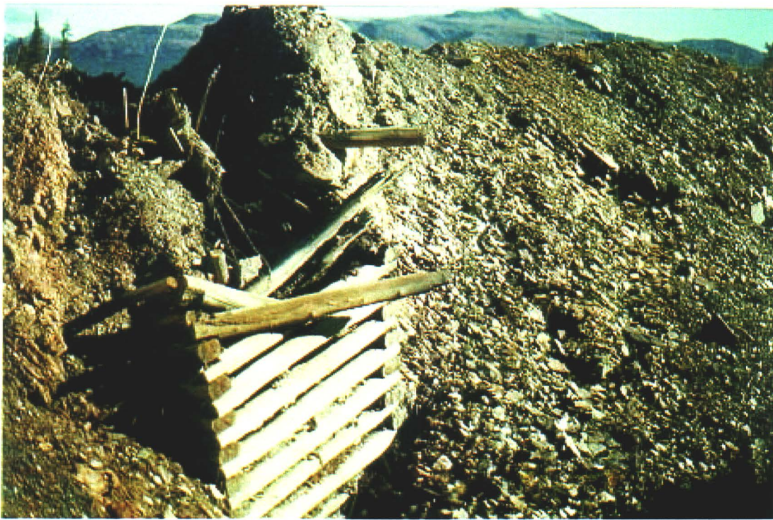
Photo 59-2. Collapsed shaft in center of trench.
