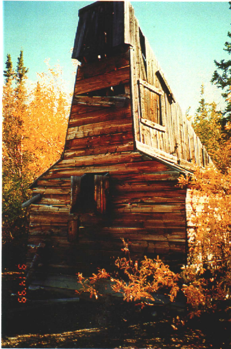
Photo 61-4: Wood framed headframe (61A).
