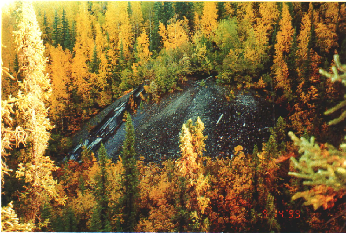
Photo 61-2: Waste rock and loadout structure below adit.
