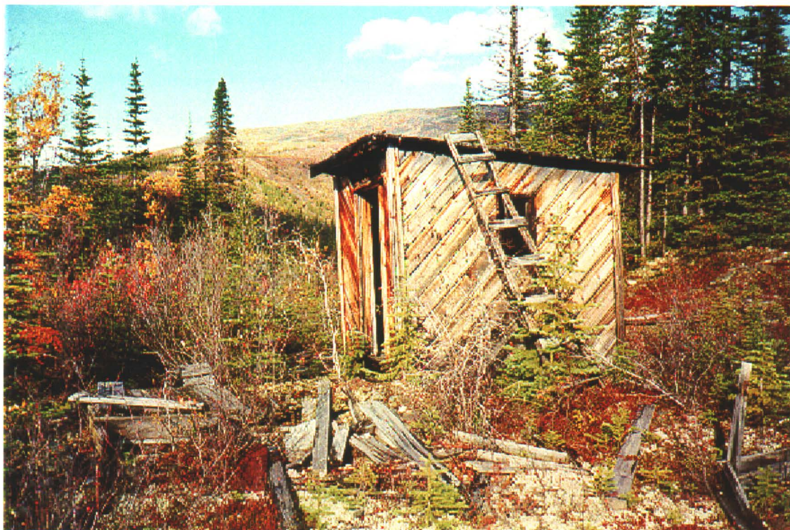
Photo 71-5: Mine shed (Bldg. 71-1). (Azimuth 000°)
