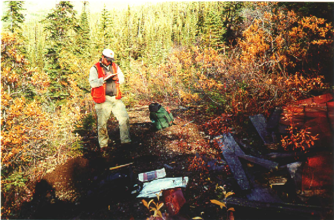
Photo 71-3: Waste rock dump below shafts A01 and A02. Note natural revegetation. (Azimuth 040°)
