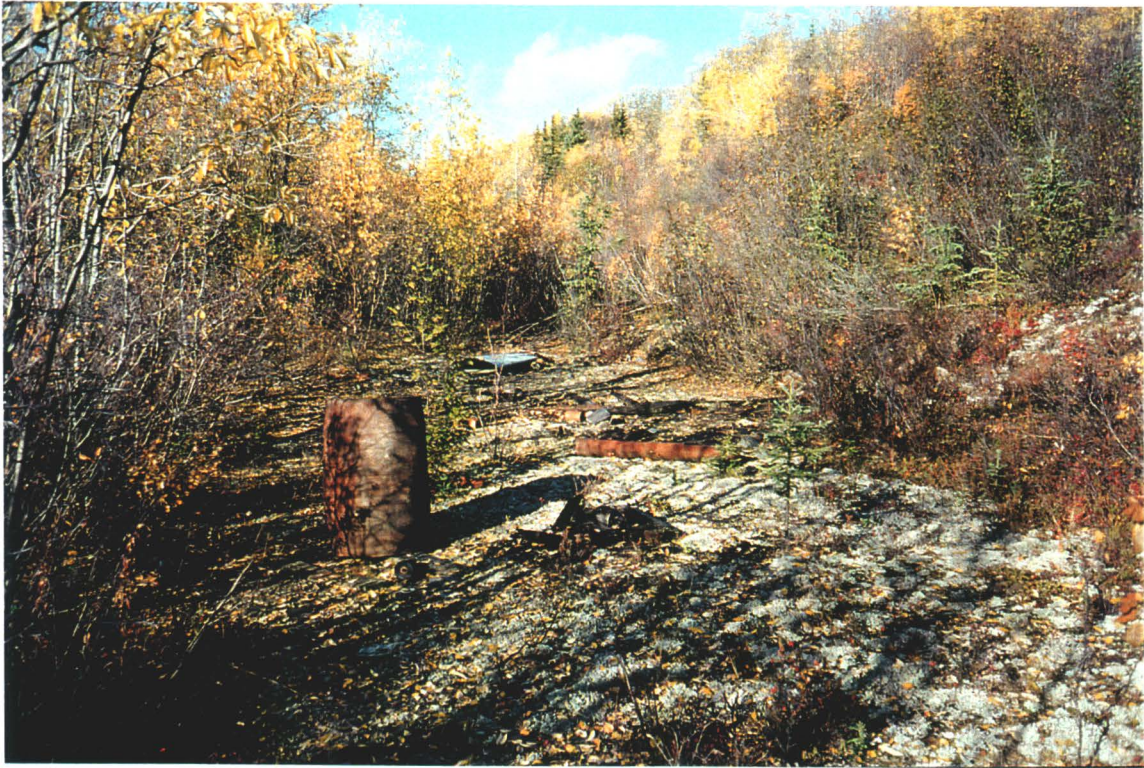
Photo 72-6: Levelled mine portal area showing metal and wood debris.
