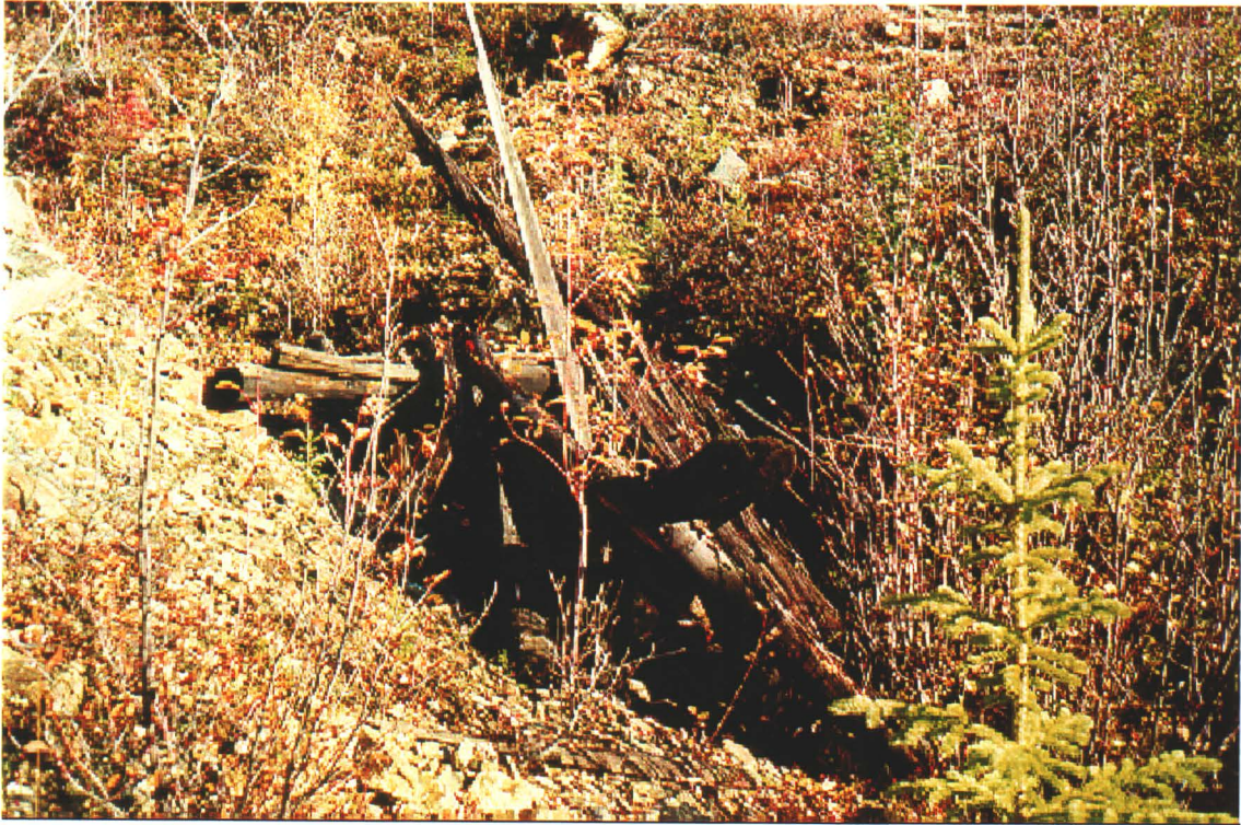
Photo 72-1: Collapsed adit Ironclad portal. (Azimuth 000°)
