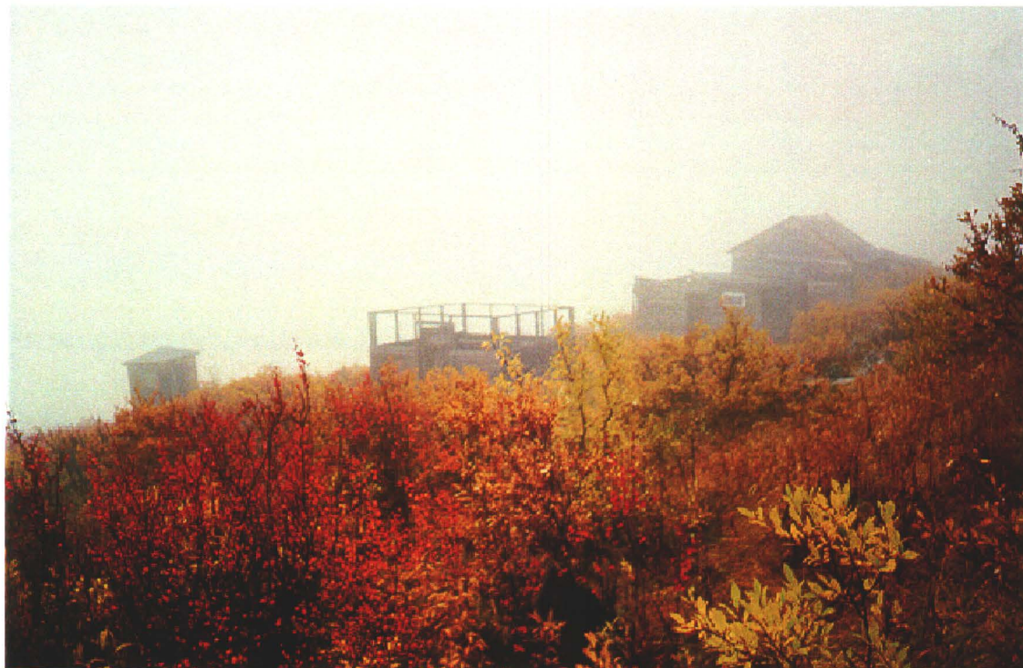
Photo 73-5: Overview of Gambler camp buildings. No changes noted since 1996 inspection. (Azimuth 130°)
