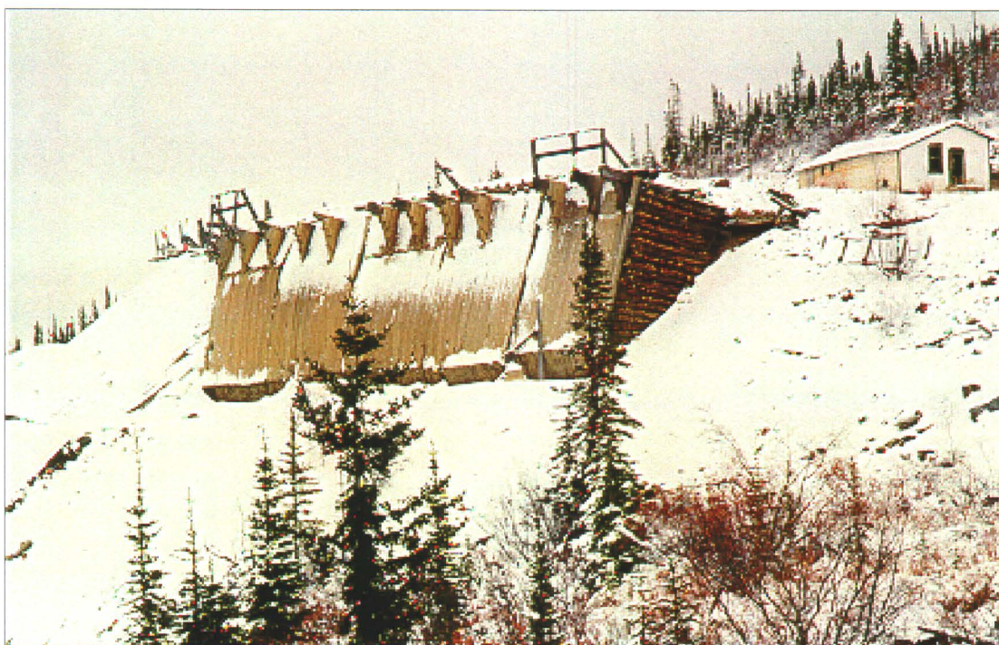
Photo 76-2: Timber retaining structure for the loading area.
