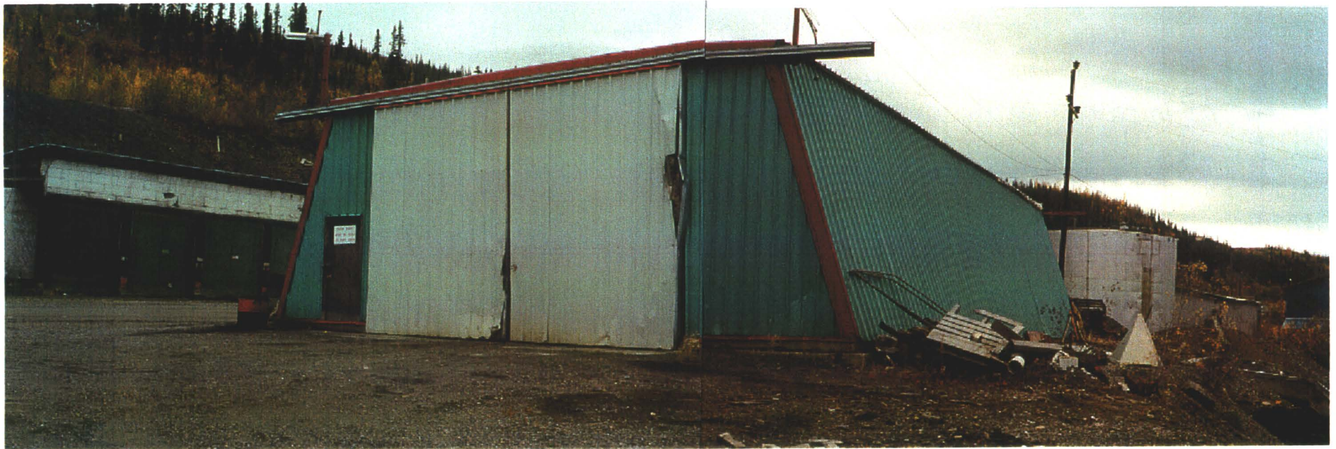
Photo 78-19 : Elsa. The large aqua-coloured building is the Machine Shop (Building #24), the light machine shop is to the left. (Azimuth 170°)
