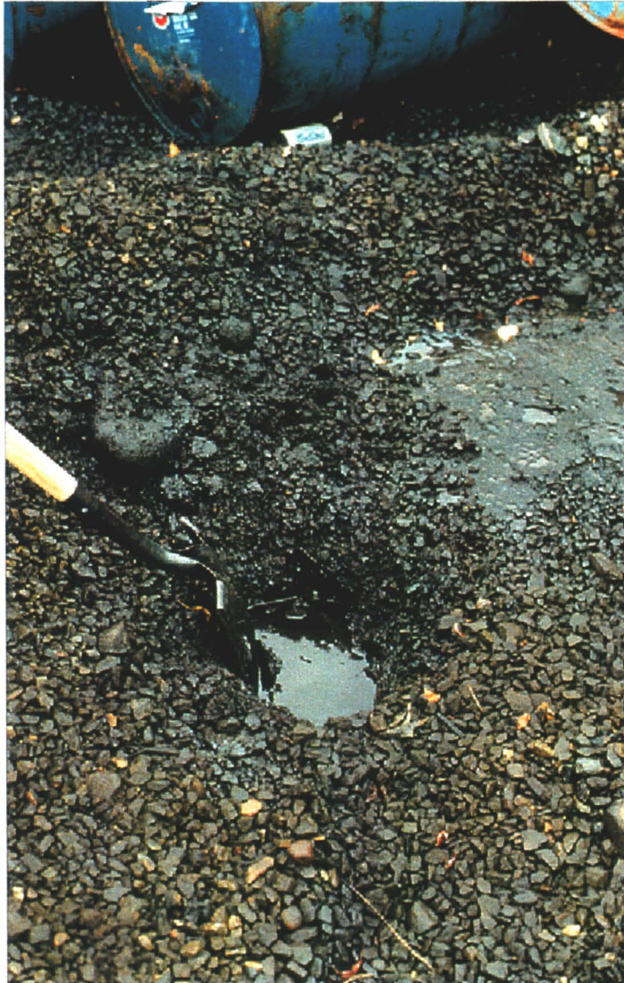
Photo 78-46 : Elsa. At Waste Fuel Storage Area #1 a small test pit revealed that the gravel was saturated with oil to at least 40cm. (Azimuth 350°)
