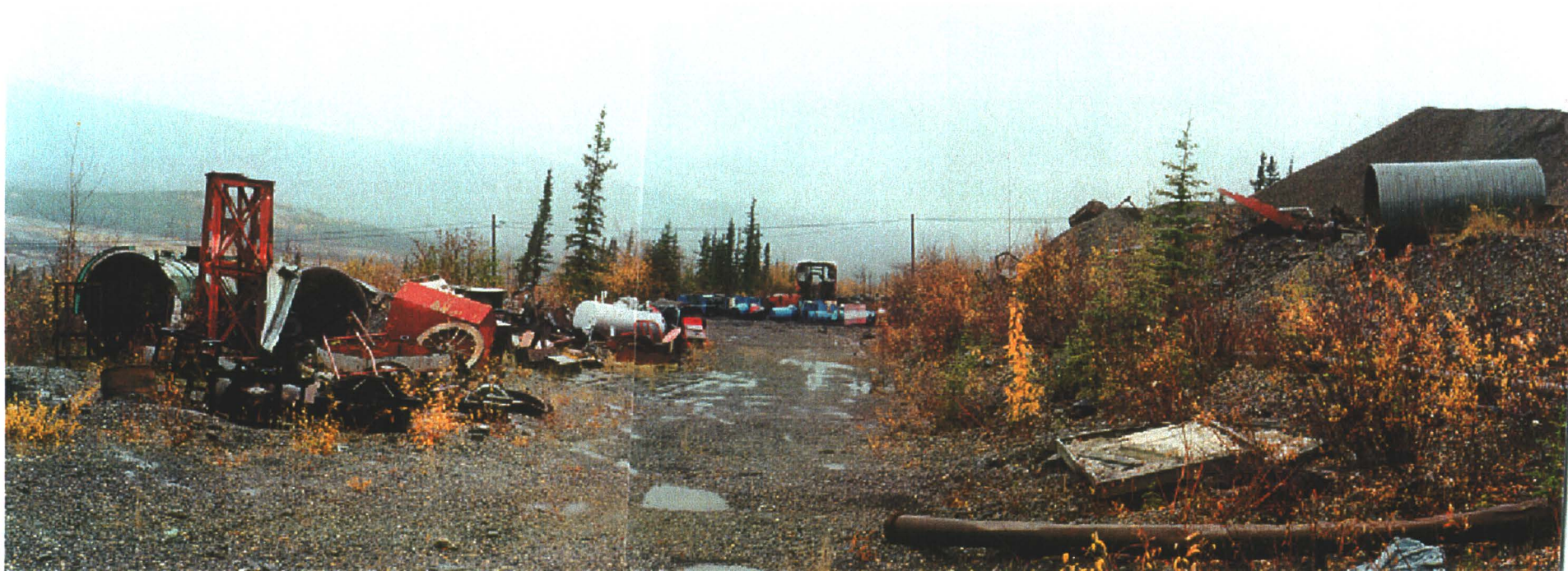
Photo 78-59 : Elsa. Solid Waste Dump Area #6. This dump is mostly scrap metal and is located just downhill of the Mill, beside Hwy #2. (Azimuth 040°)
