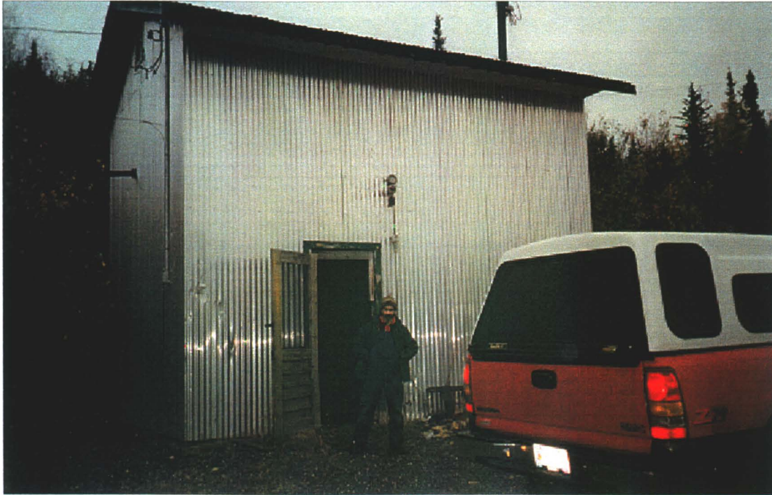
Photo 78-36 : Elsa. Town water supply pump house. (Building #53)
