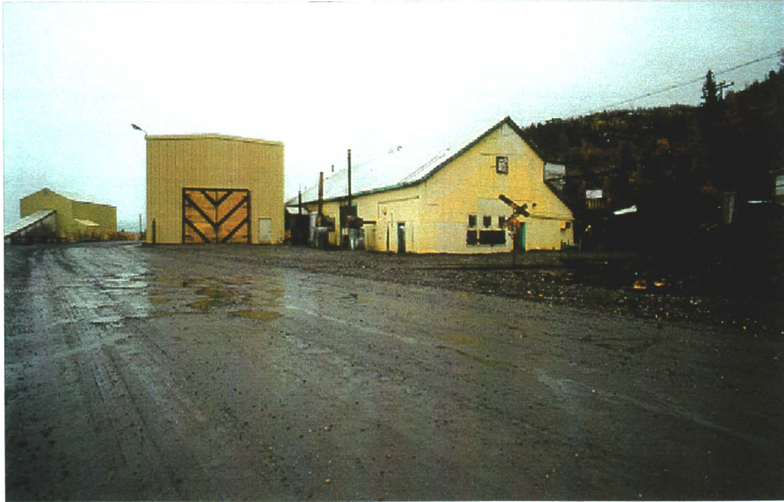
Photo 78-28 : Elsa. The generator building is on the right, the vehicle & heavy equipment warehouse is in the centre, and the building in the background is the crusher house. The 3 diesel exhaust stacks are visible on the left side of the generator building.
