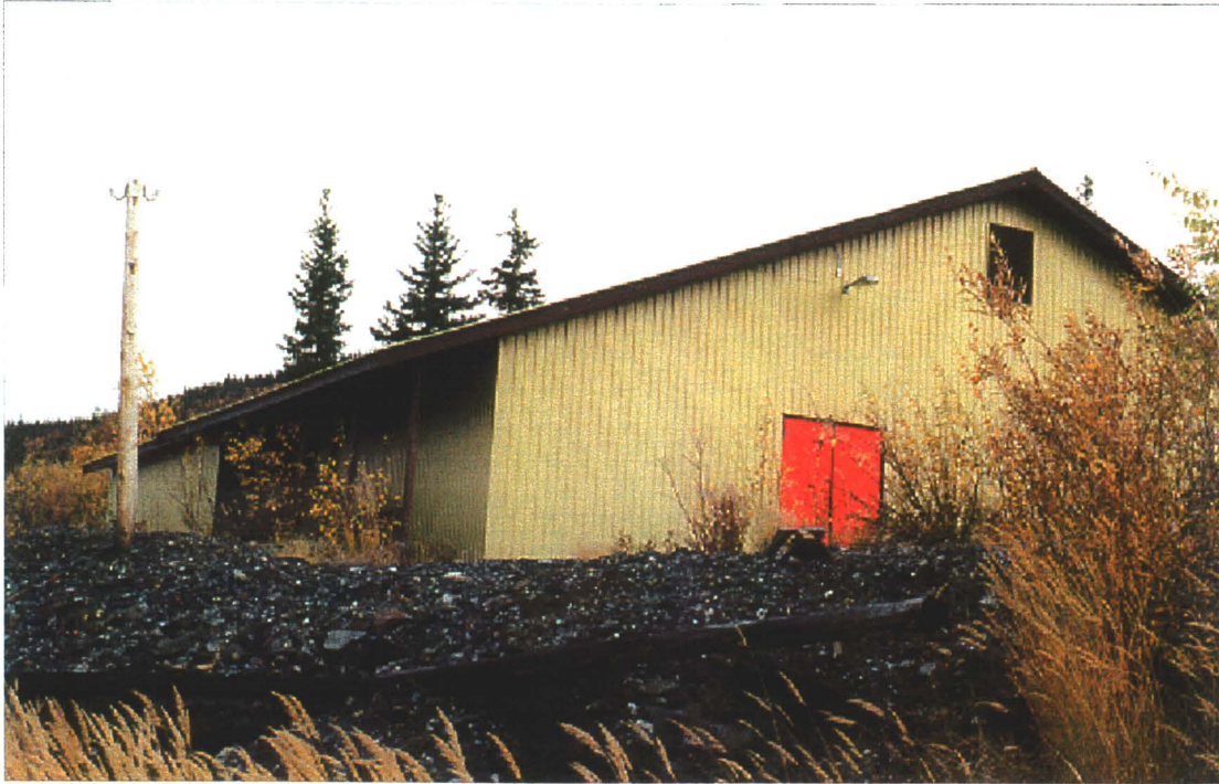
Photo 78-24 : Elsa. Building #29, the swimming pool building. (Azimuth 085°)
