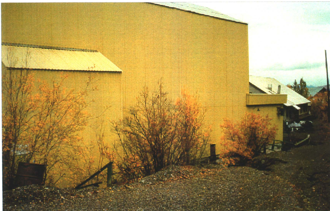
Photo 78-15 : Elsa. The yellow building on the left is the crusherhouse, (Building #20); the light brown building on the right is the assay lab (Building #37).
