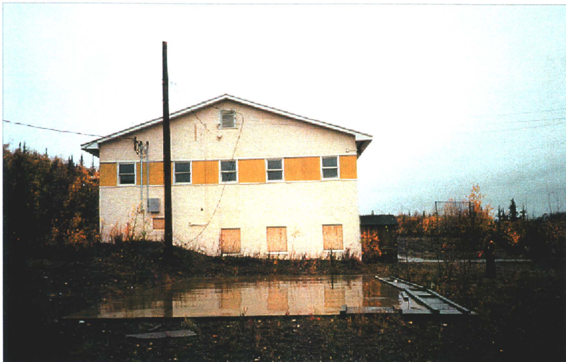
Photo 78-43 : Elsa. Elsa school. Note black underground fuel storage tank stand pipe at right side corner. (Azimuth 210°)
