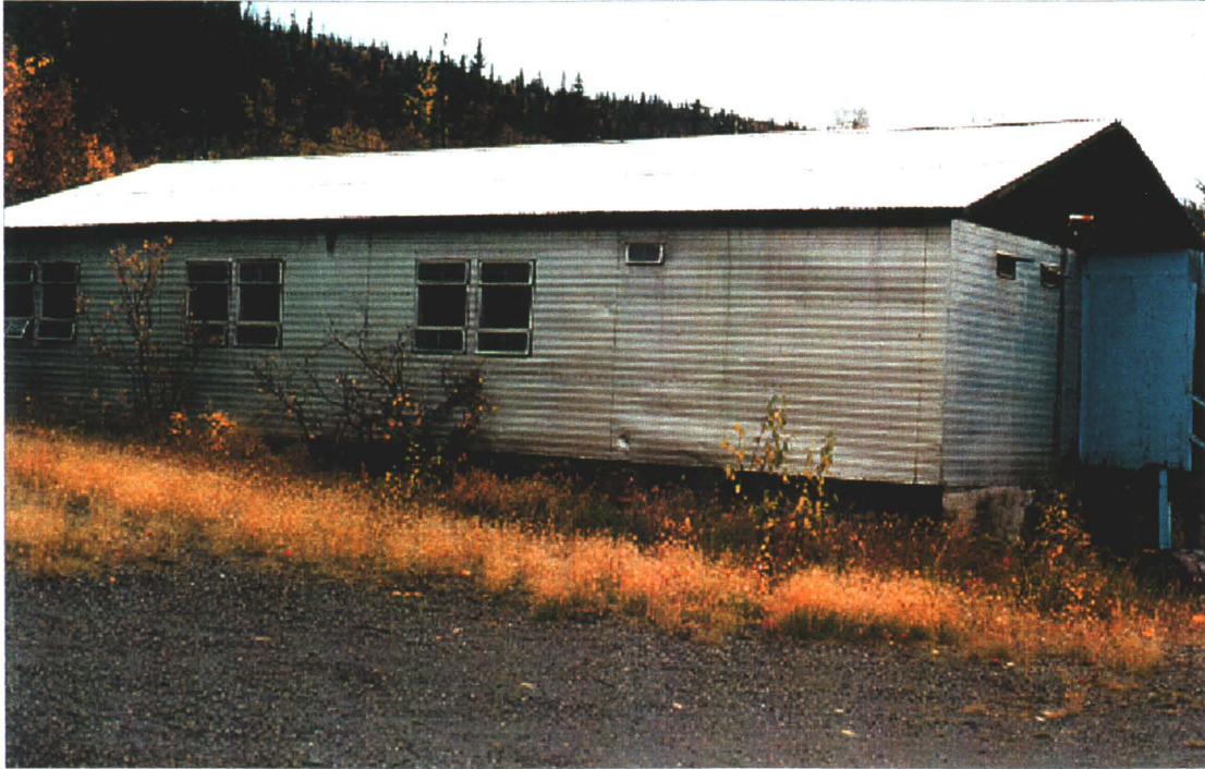
Photo 78-10 : Elsa. Building #14, the Union Shop. (Azimuth 200°)
