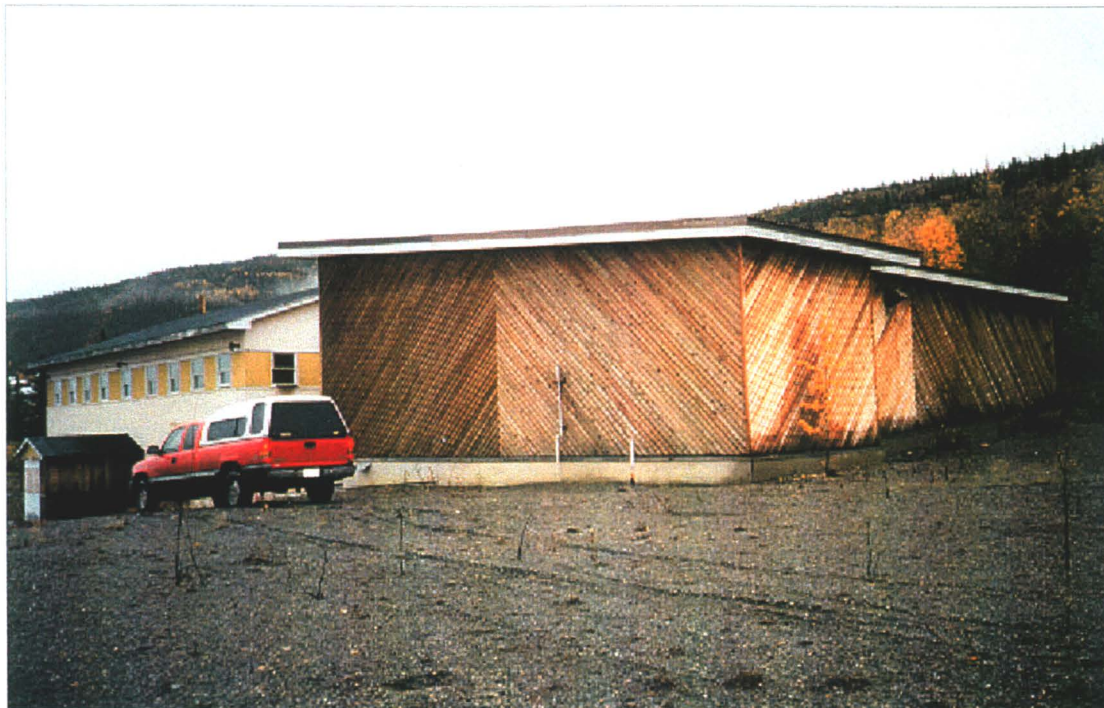
Photo 78-37 : Elsa. Elsa school. Note white probable underground fuel storage tank stand pipes at nearest corner. (Azimuth 090°)
