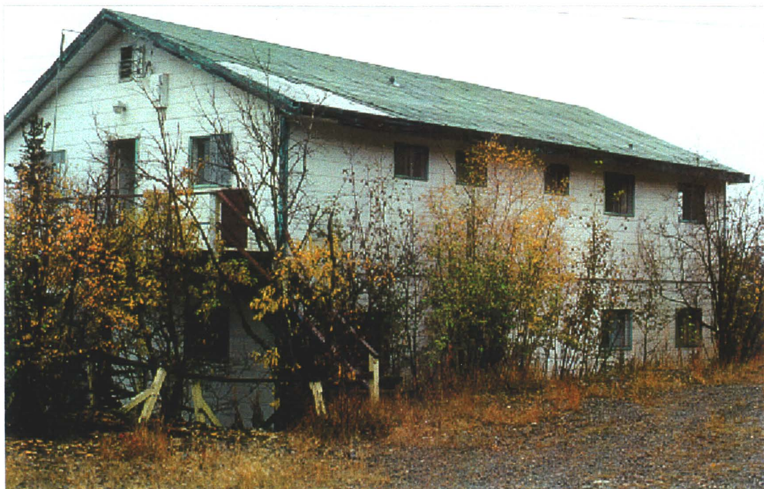
Photo 78-31 : Elsa. Building #41, a two-story apartment complex. (Azimuth 360°)
