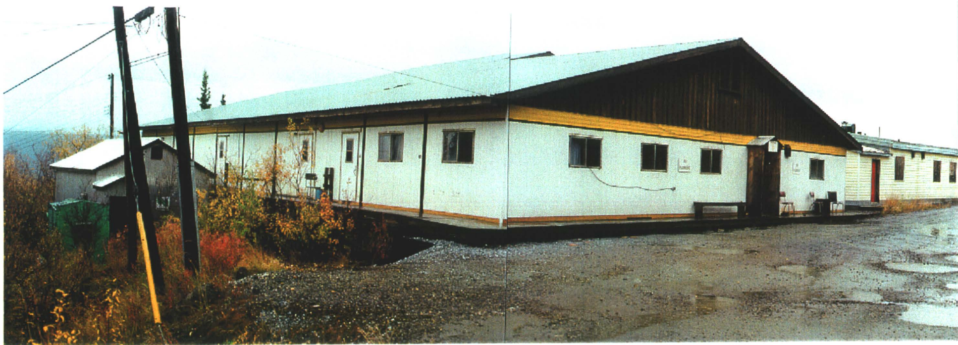
Photo 78-13 : Elsa. Building #18, the Norwest Tel Hut, is the corrugated steel building on the left, and the Dry / Change Building is on the right. (Azimuth 350°)
