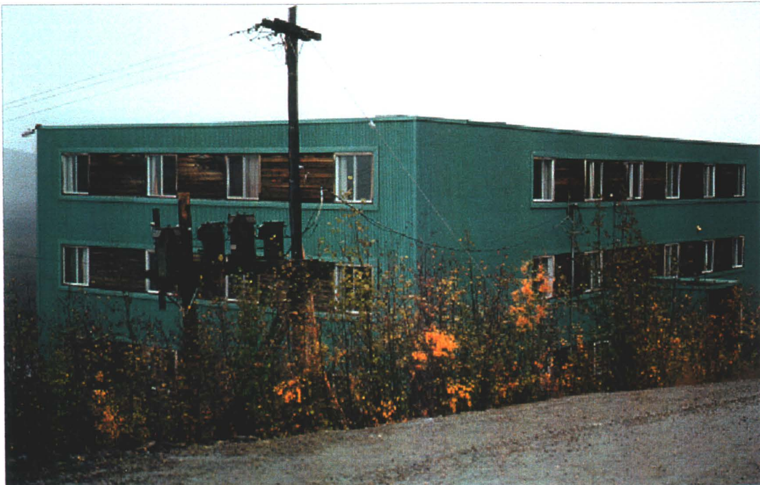
Photo 78-5 : Elsa. Building #7 is one of the newer bunkhouses. Note transformers in the foreground. (Azimuth 010°)
