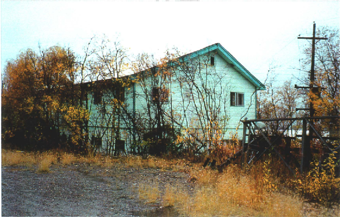
Photo 78-30 : Elsa. Looking west at the Men's Staffhouse (Building #39). (Azimuth ~270°)
