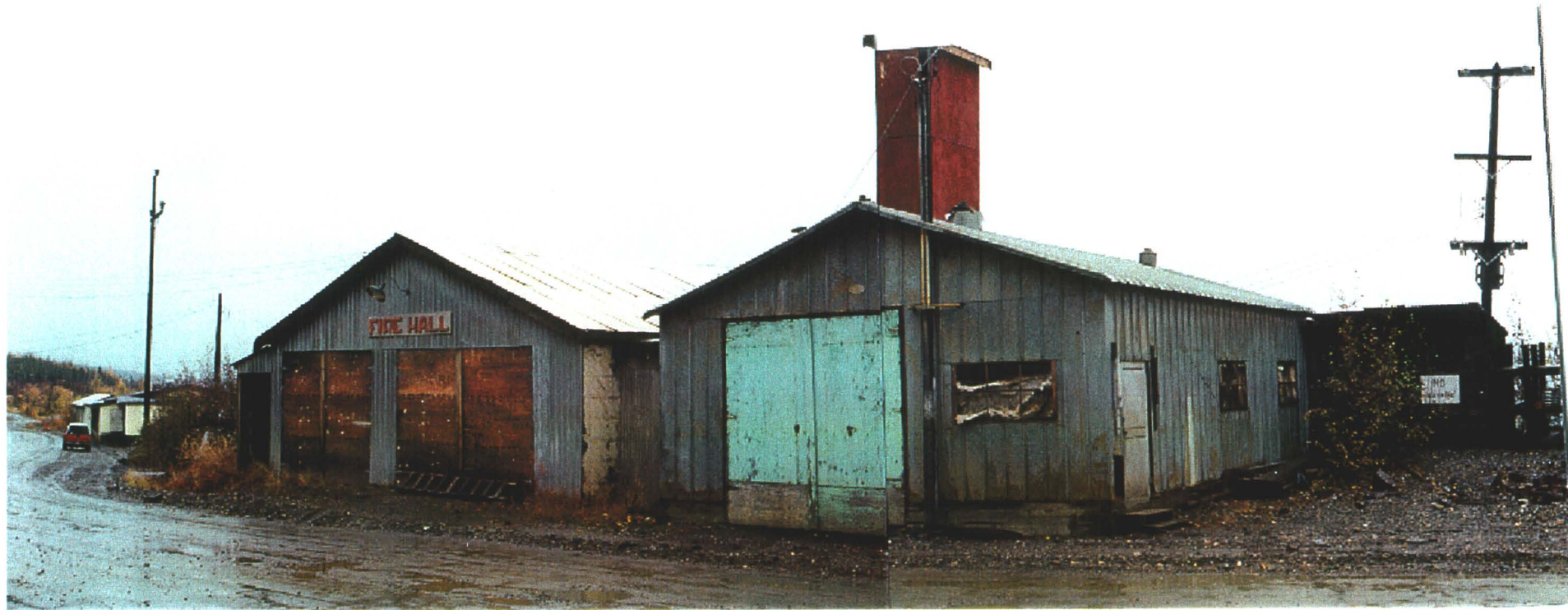
Photo 78-27 : Elsa. Building #33, the Fire Hall is on the left of the photo and Building #34, possibly the dry change house, is on the right. (Azimuth 260°)
