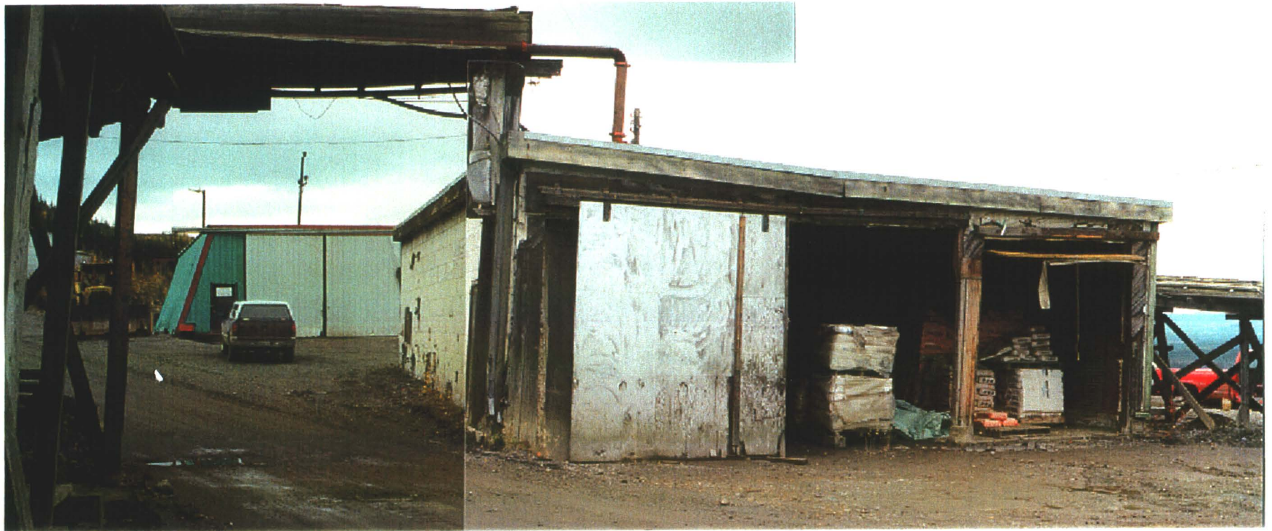
Photo 78-18 : Elsa. Building #23, the No.2 Garage, is in the foreground, the Machine Shop (Building #24) is in the background. (Azimuth 260°)
