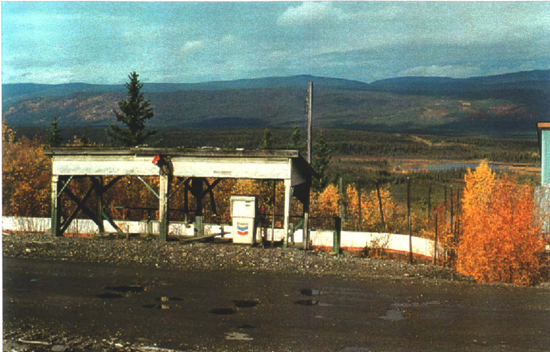
Photo 78-23 : Elsa. Fuel Storage Area #2, a single Chevron pump, located uphill from the skating rink. (Azimuth 030°)
