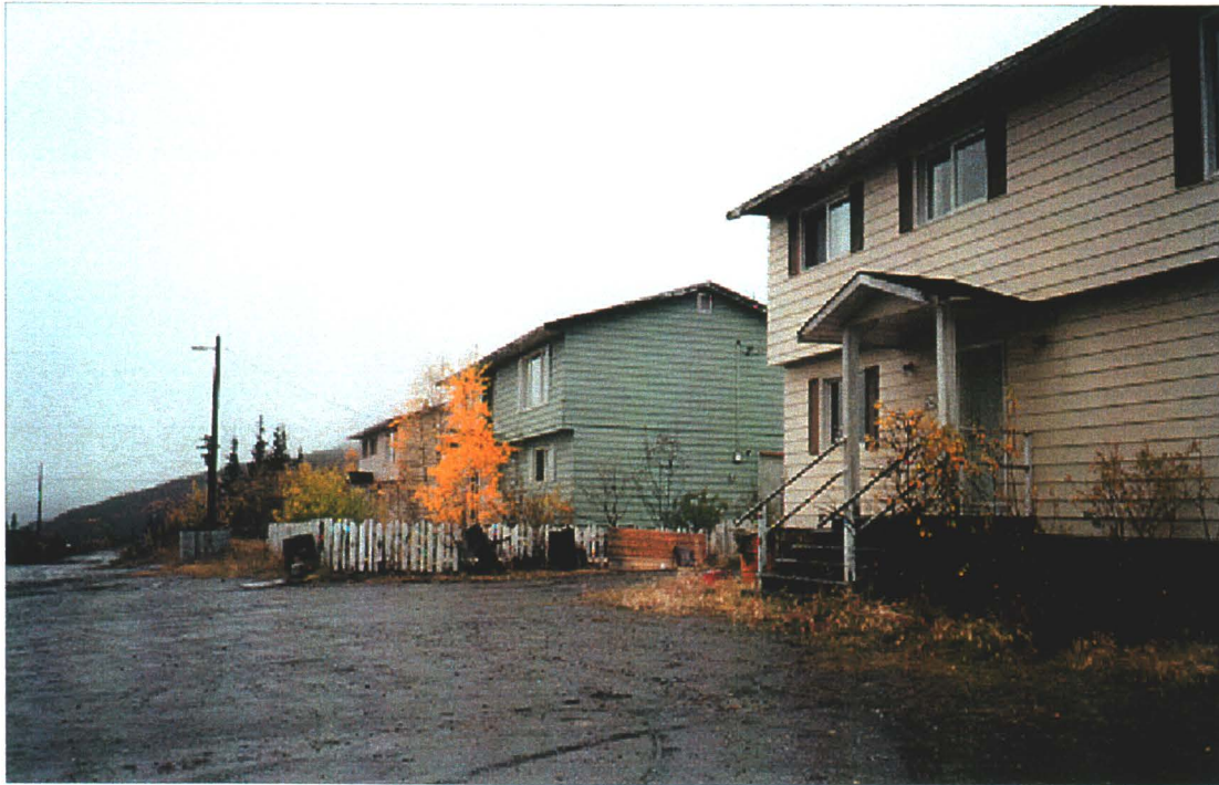
Photo 78-34 : Elsa. Occupied mine houses. (Buildings #44 - 51)
