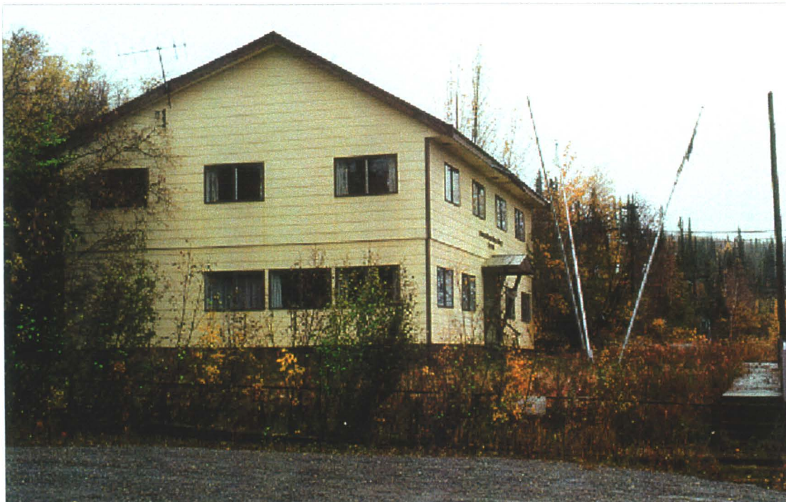
Photo 78-29 : Elsa. The Administration Building (Building #38) is located to the southeast of the floatation mill. (Azimuth 190°)
