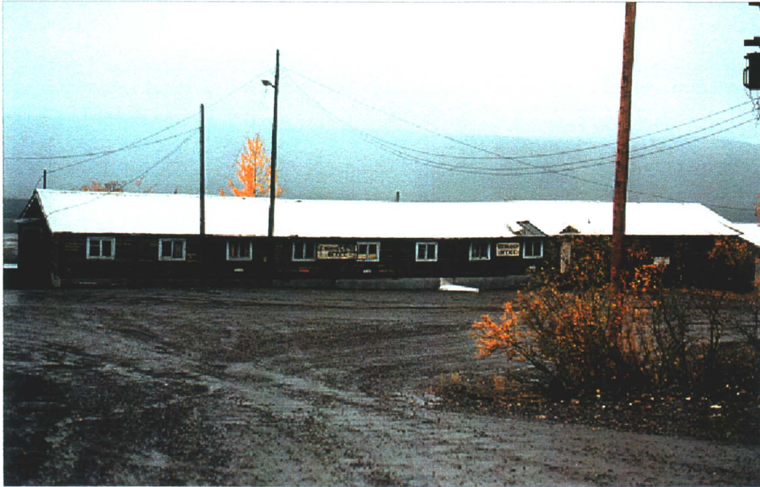
Photo 78-6 : Elsa. Building #8 is the geology and engineering offices. (Azimuth 340° )
