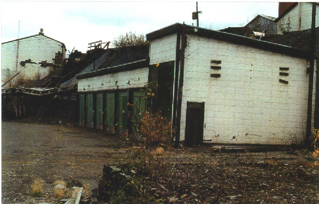
Photo 78-20 : Elsa. Building #25, Light Vehicle Shop is in the foreground, with Building #51, the crusherhouse, in the background. (Azimuth 060°)
