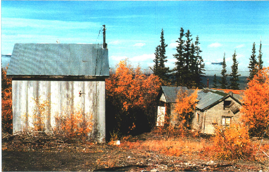
Photo 78-38 : Elsa. View of buildings in the Flat Creek area, the water pump building (Building #55) is on the left and residence #1 (Building #56) is on the right. (Azimuth 350°)
