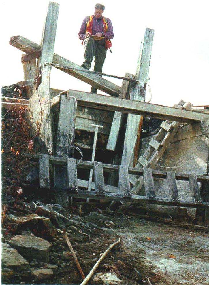
Photo 79-9. Decant in Dam No. 2, upstream side.
