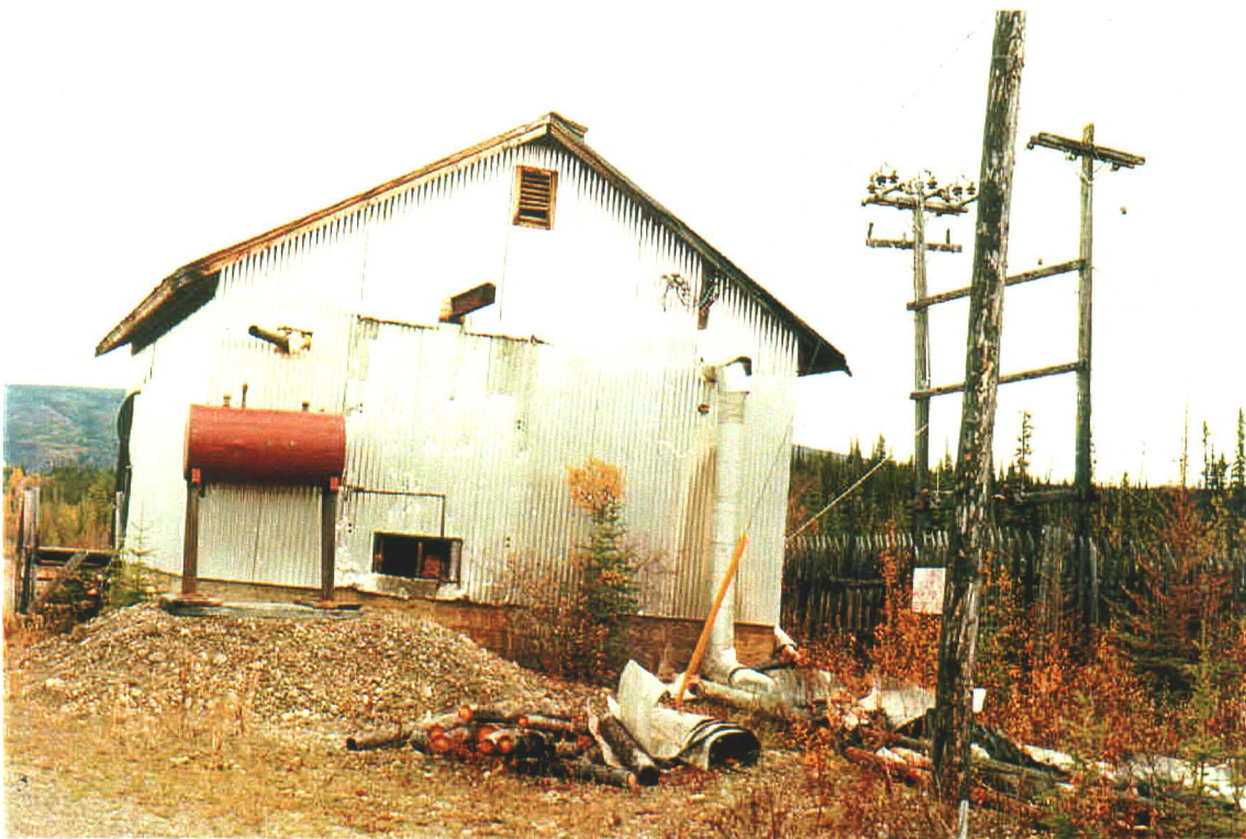
Photo 79-23. Pressure pump house that pumps the fresh lake water to the Elsa townsite. Note picket fence to the right of the house that contains the transformer that is in use.
