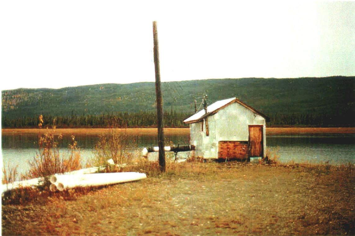
Photo 79-22. Pump house on unnamed lake that is the fresh water supply for the Elsa townsite.
