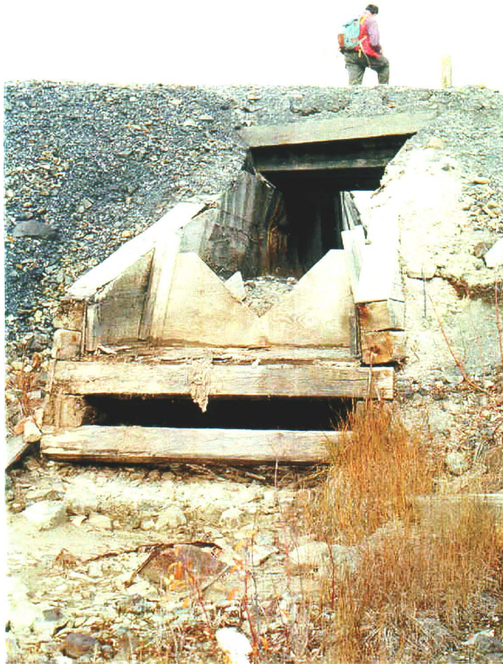
Photo 79-10. Decant in Dam No. 2, downstream side. Note lime precipitate around decant.
