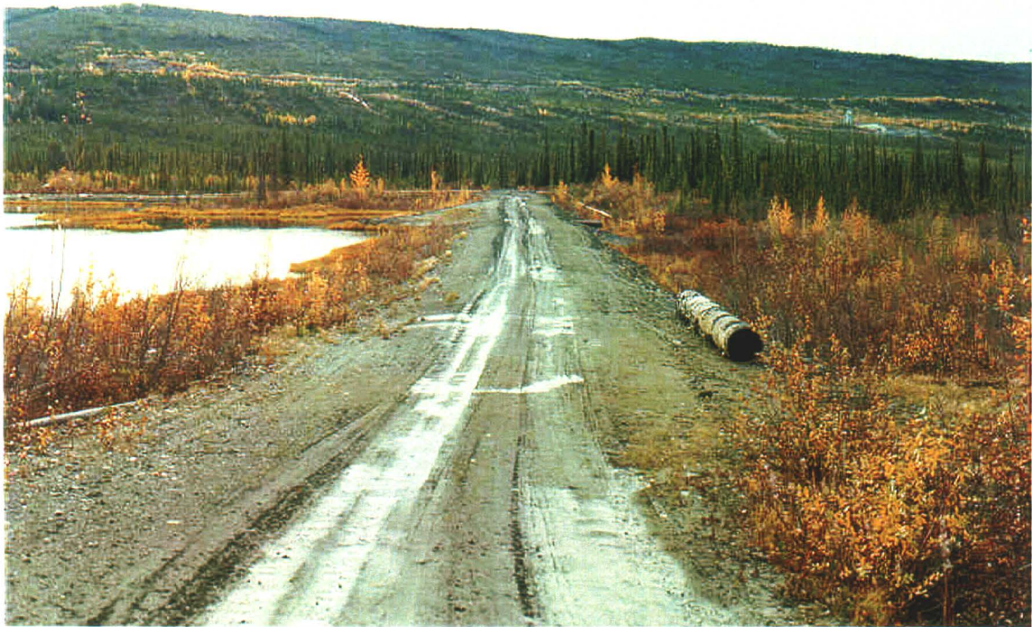
Photo 79-11. Tailings Dam No. 3, looking south.
