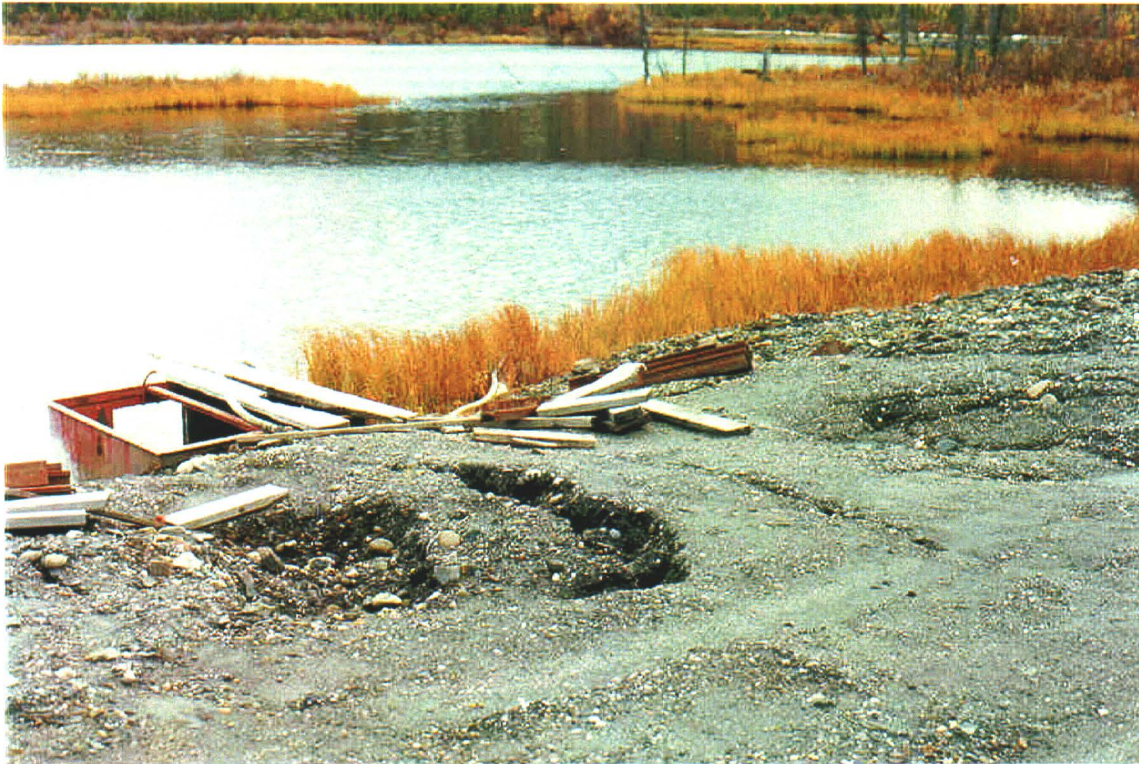
Photo 79-13. Wooden decant and v-notch weir in Dam No. 3. Note subsidence around decant.
