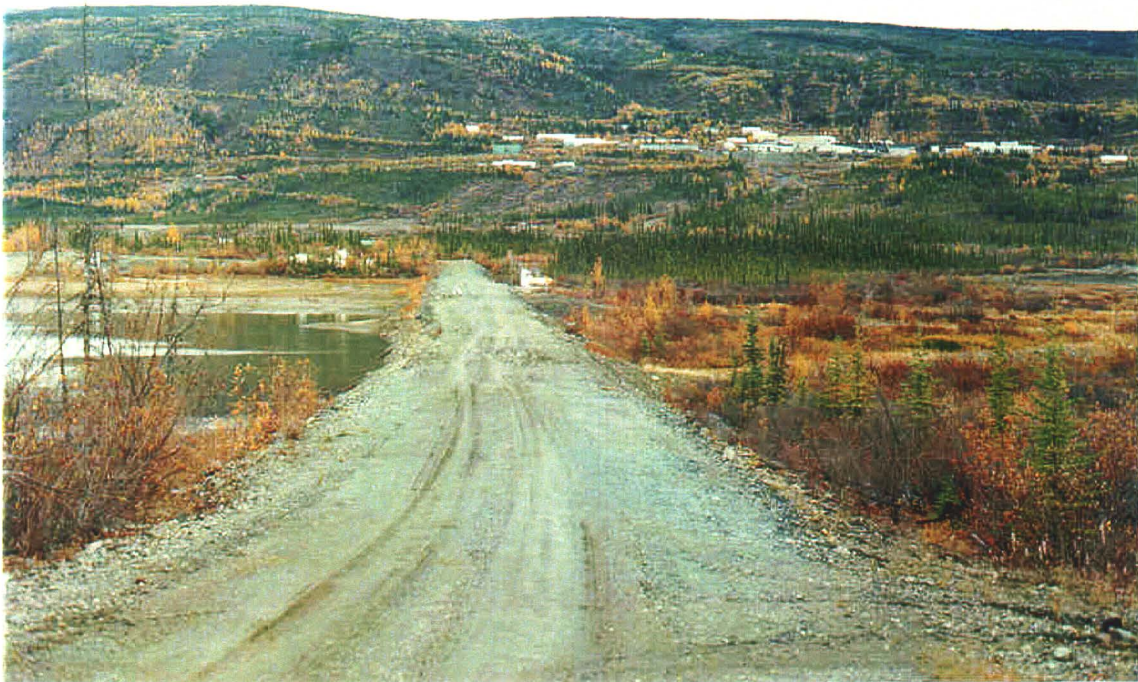
Photo 79-5. Tailings Dam No. 2, looking southeastward. The lime treatment plant can be seen at the far end of the dam. The Elsa townsite is in background on the hill.
