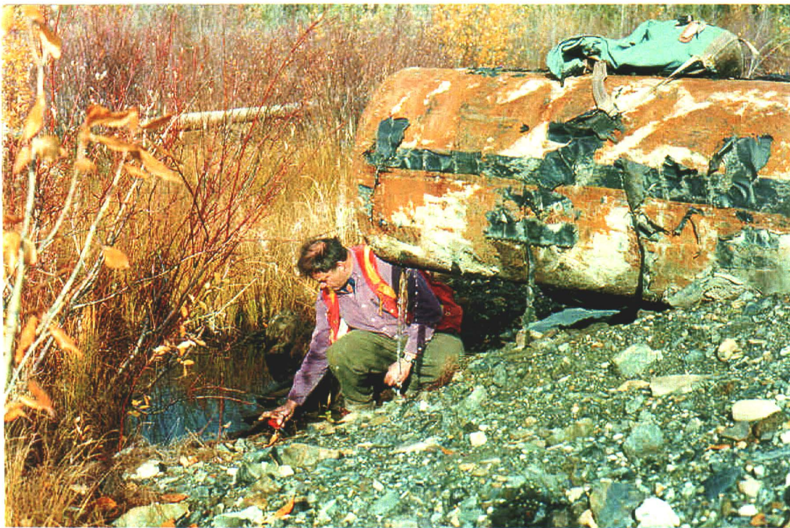
Photo 79-13. Wooden decant and v-notch weir in Dam No. 3. Note subsidence around decant.
