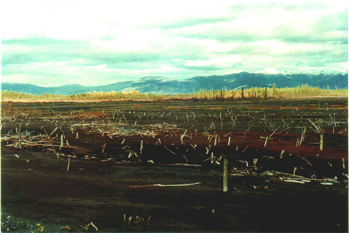
Photo 79-4. Exposed tailings behind Dam No. 1.
