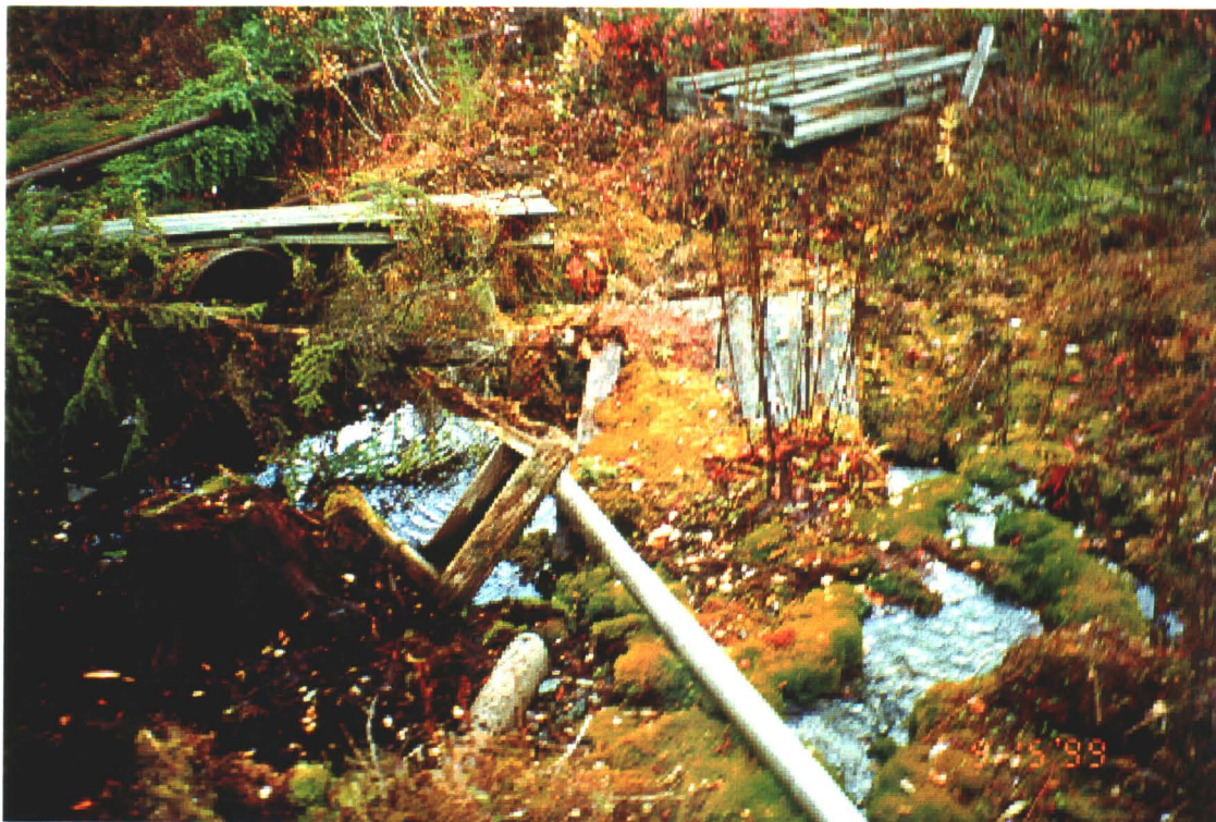
Photo 81-6: Tailings pipeline in forested area north of millsite.
