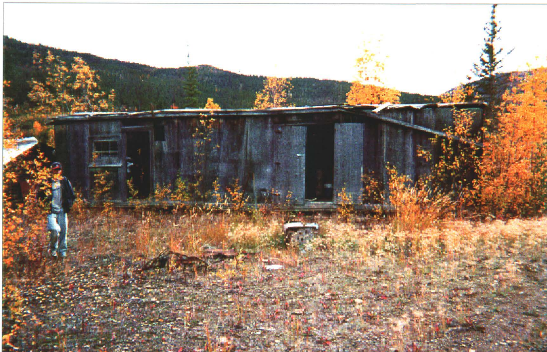
Photo 88-4 : Dublin Gulch. Exploration Camp - workshop & storage looking S.
