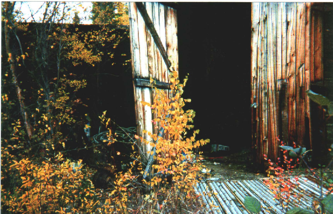
Photo 88-6 : Dublin Gulch. Exploration Camp - equipment building & garage looking N.E.
