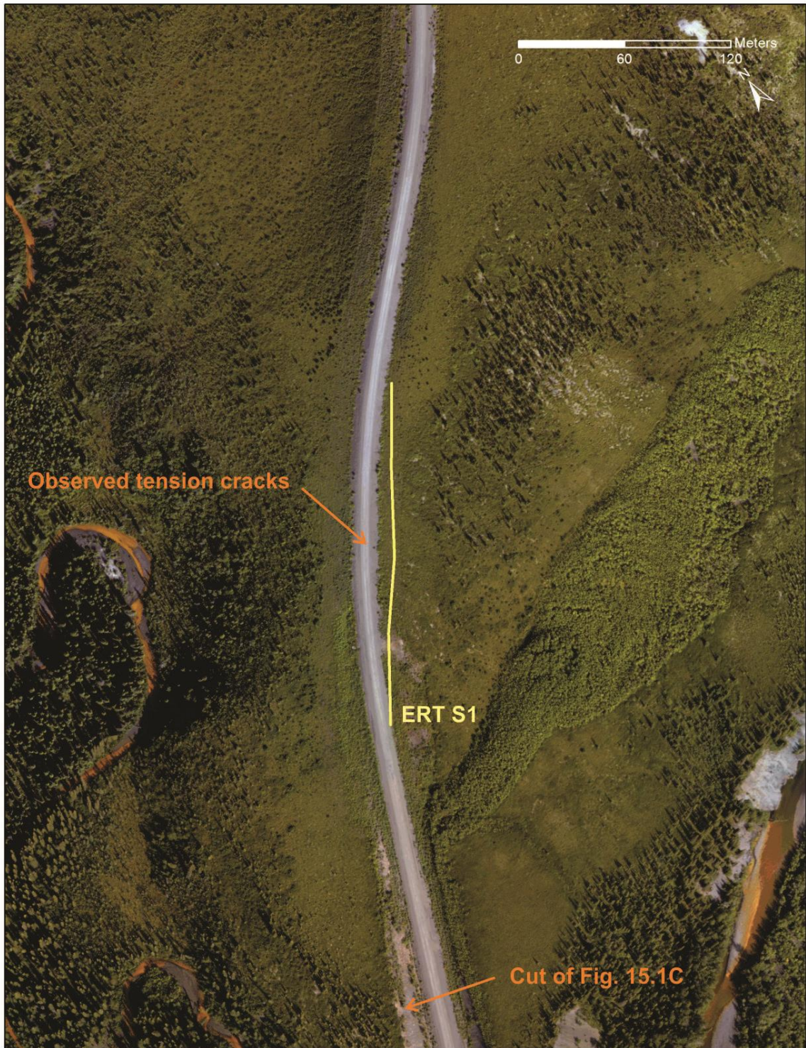
Figure 3.15.3 Aerial view of site DH447.
