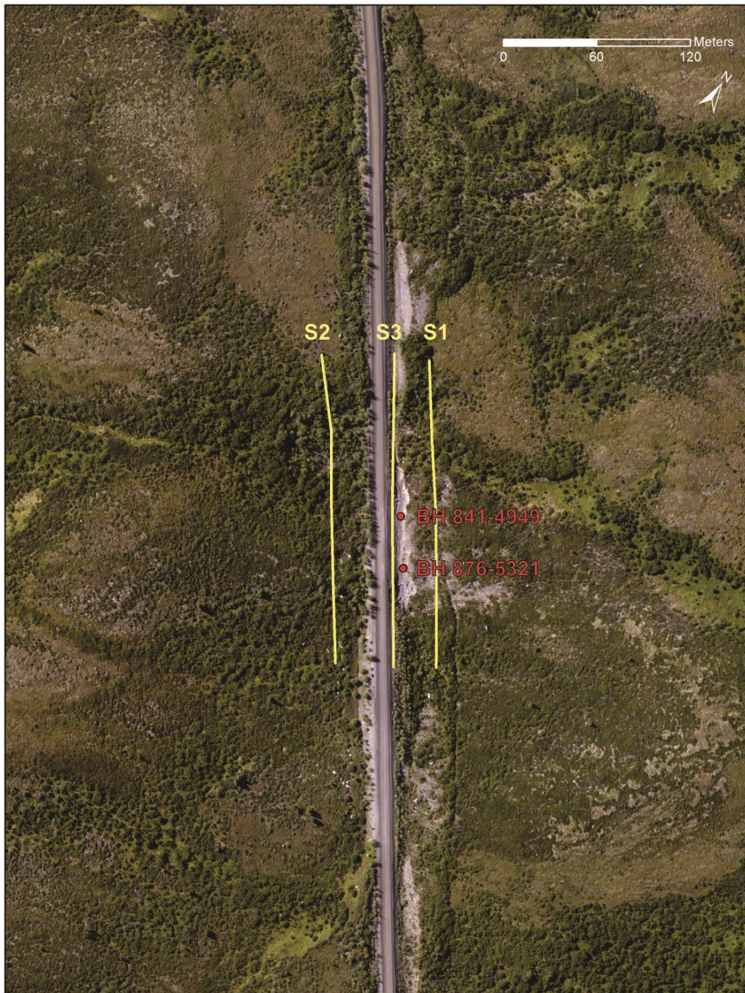
Figure 3.1.3 Aerial view of site DH82
