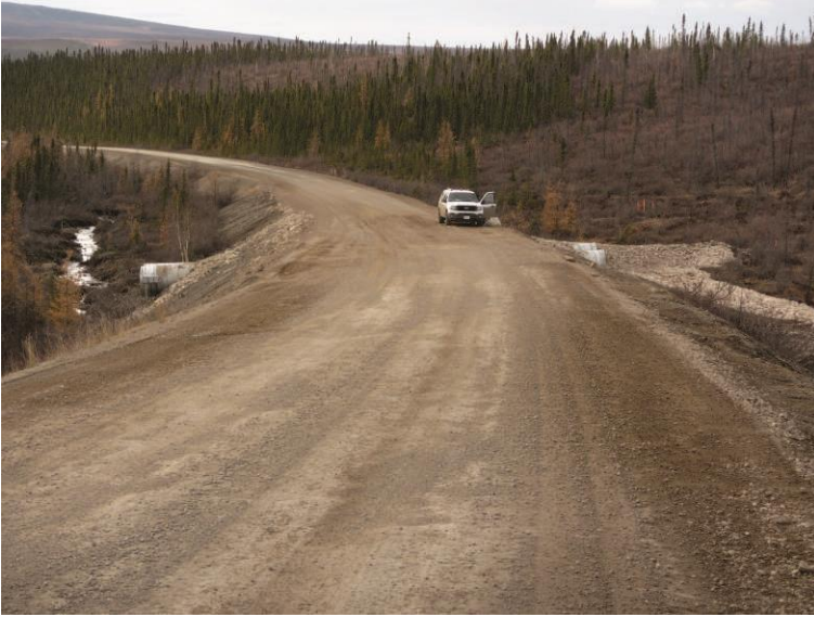
Figure 3.10.1 Culvert at site DH381.
