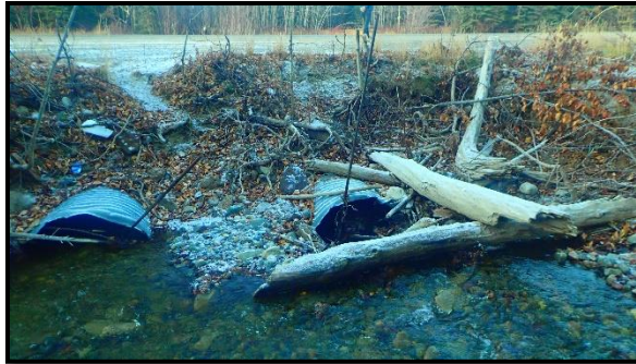
Figure 48. Head of three culverts in the Montague roadhouse rest area in October 2022 (culverts are mostly blocked by debris).
