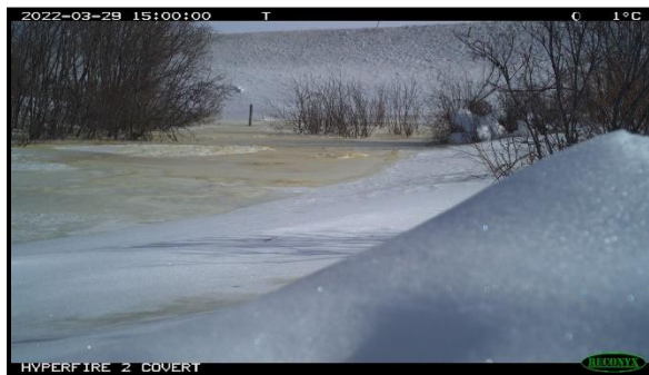
Figure 20. Slavin Creek (km 98.6) timelapse photo of culvert head buried by aufeis on March 29, 2021 (Photo provided by McMaster University, Sean Carey's research team).
