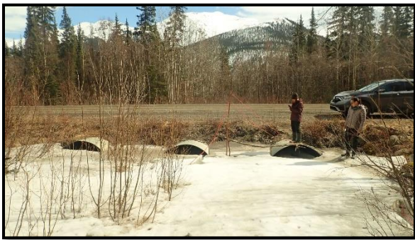
Figure 13. Yin Tang Creek culvert heads on May 8, 2022.
