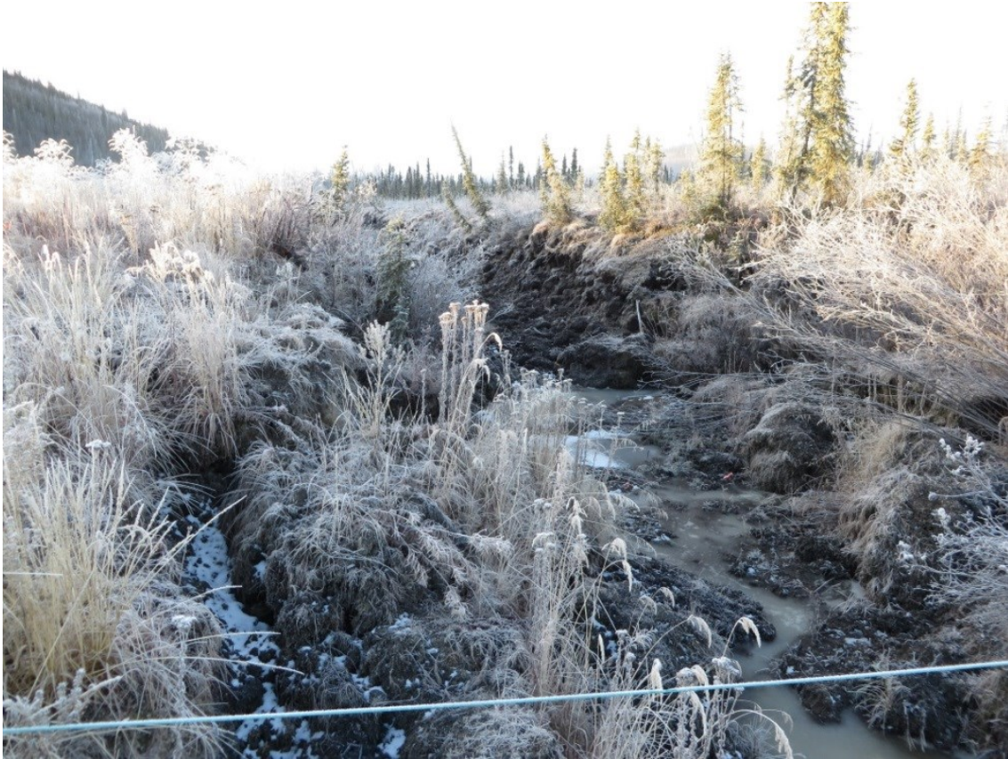
Figure 4.6.11. Thermal erosion in the ditch, facing southwest.
