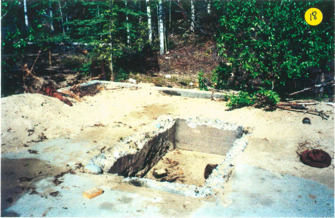
3.18: Mechanics Pit at Carcross Pump Station Site
