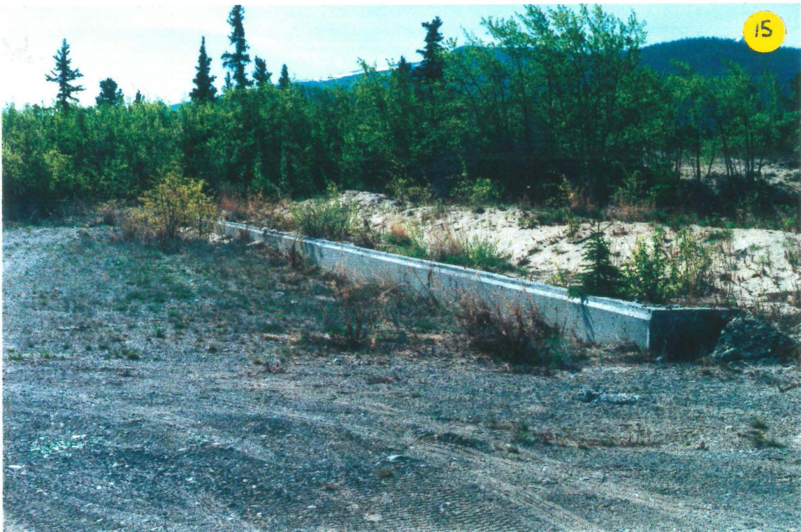
3.15: Remnants at Carcross Pump Station Site
