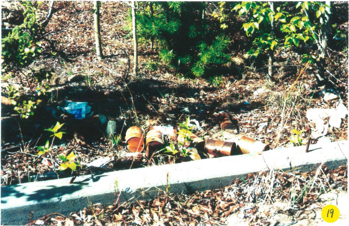
3.19: Debris at Carcross Pump Station Site
