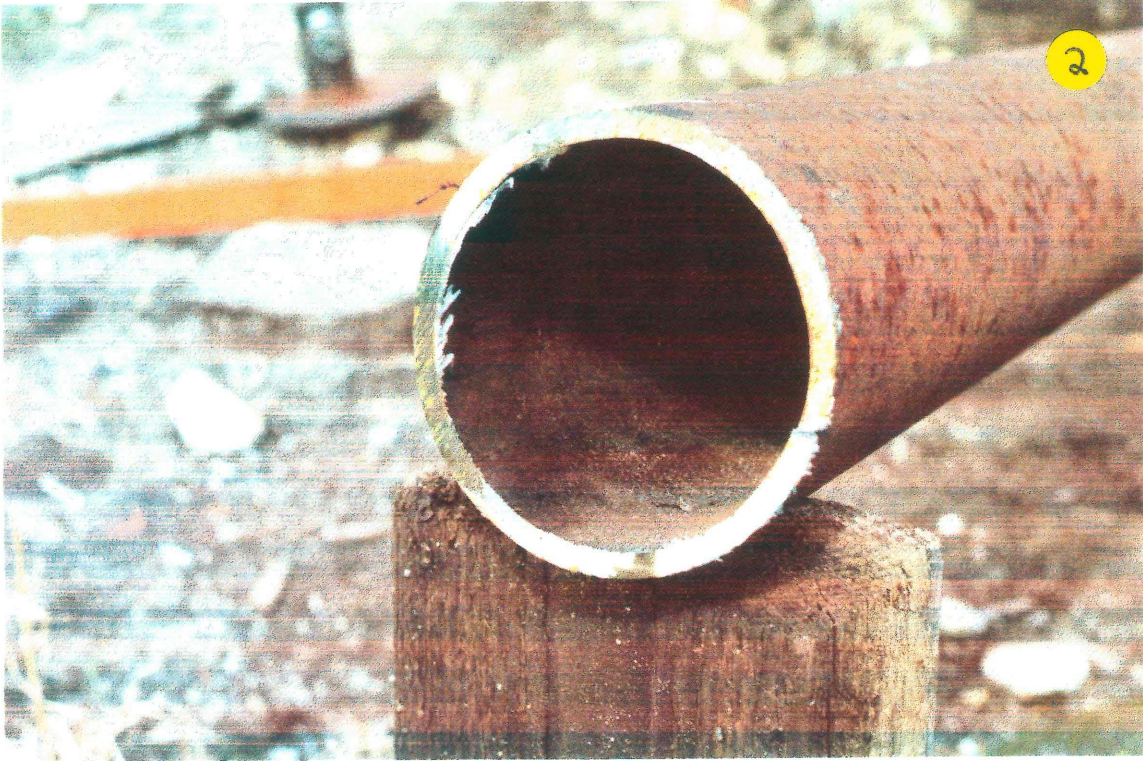
3.2: Inside Surface of Pipeline
