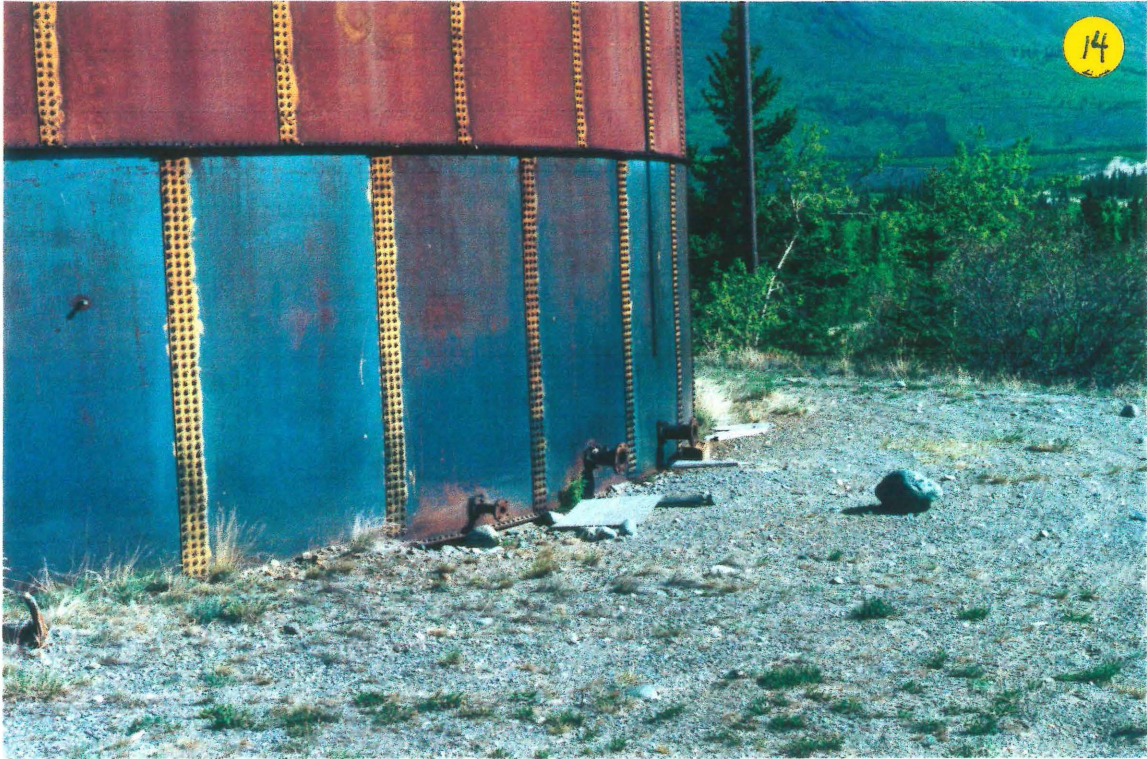
3.14: Tank at Carcross Pump Station Site
