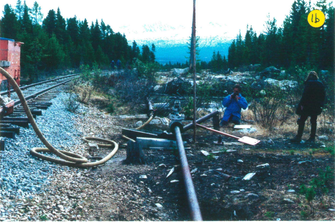
3.1b: Pig Launching Assembly
