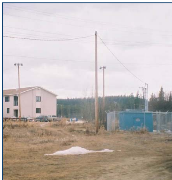
A well for drinking water extraction from the Selkirk field, in the Riverdale Area.
