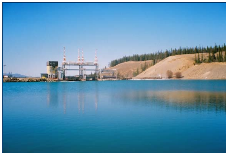
The Yukon Energy Corporation Dam, built in 1959, converted the historically significant White Horse Rapids into Schwatka Lake.
