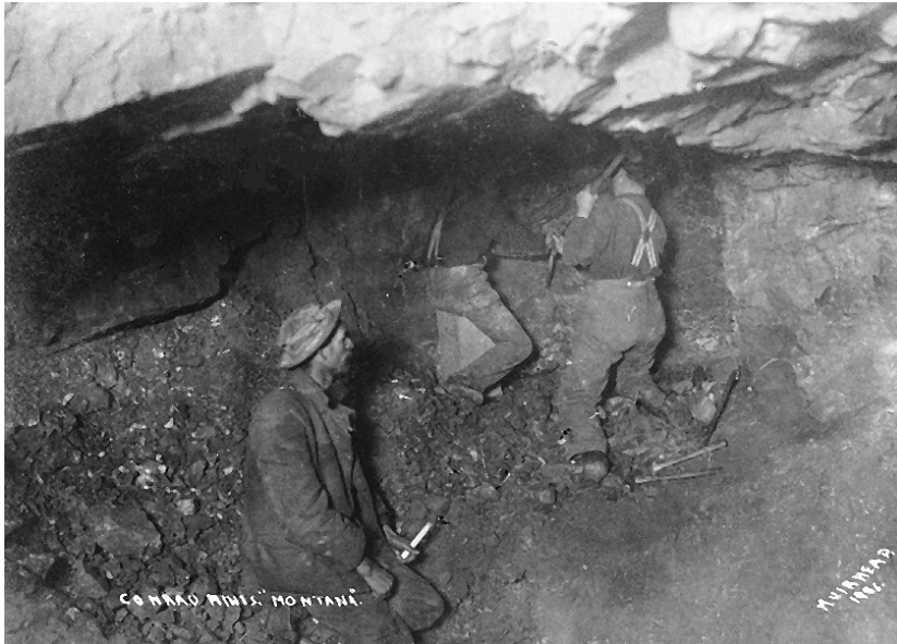
Driving tunnels at the Montana mine the hard way: a candle for light, and handtools and muscle to move tons of rock surrounding the silver ore.
