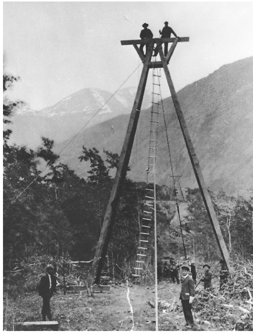
Construction of the first of the Mountain Hero tramway towers, in August 1905. Fifty men worked on the project, under the direction of R.E.Lanyon, of Nelson, British Columbia. This photo, by Case & Draper, was also produced as a postcard.
