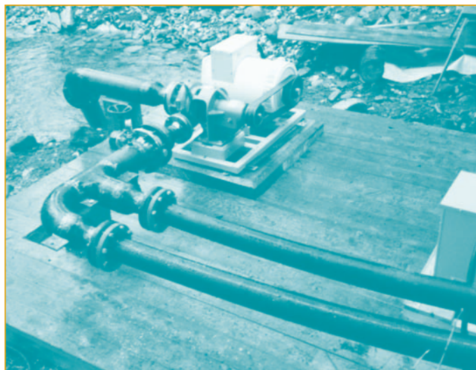
Figure 18. Pump-as-turbine with 12-kW output using twin 10-cm (4-in.) penstock (photo courtesy of Thompson and Howe Energy Systems Inc.)
