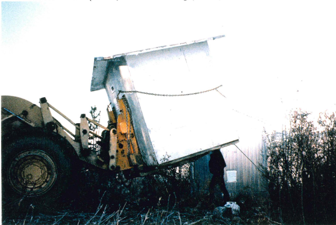
Photo B: Old building being moved
