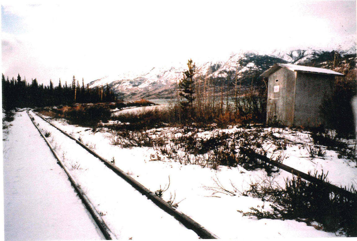
Photo I: View of site with rail line and pipe line
