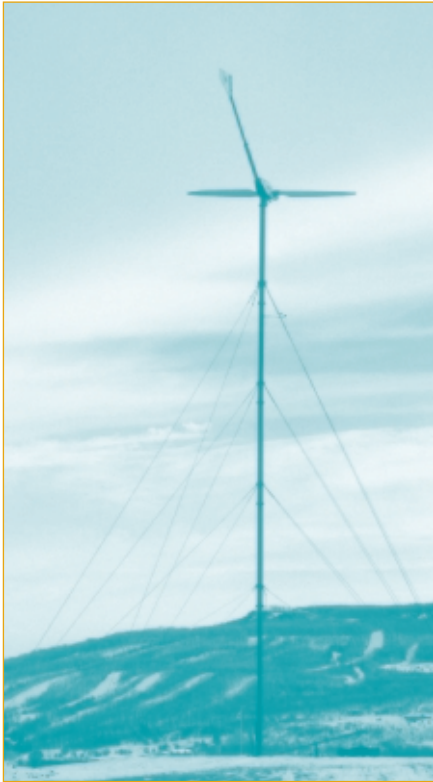
▲ Figure 9. A small 25kW Wenvor-Vergnet wind energy system in Collingwood, Ontario, supplies electricity to a rural residence. (Photo courtesy of Wenvor Technologies Inc.)
