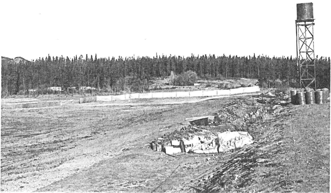
6. Site preparation complete - organic material spread, surface rototilled and seeded; water tank, 1300 l, for composting and irrigation.
