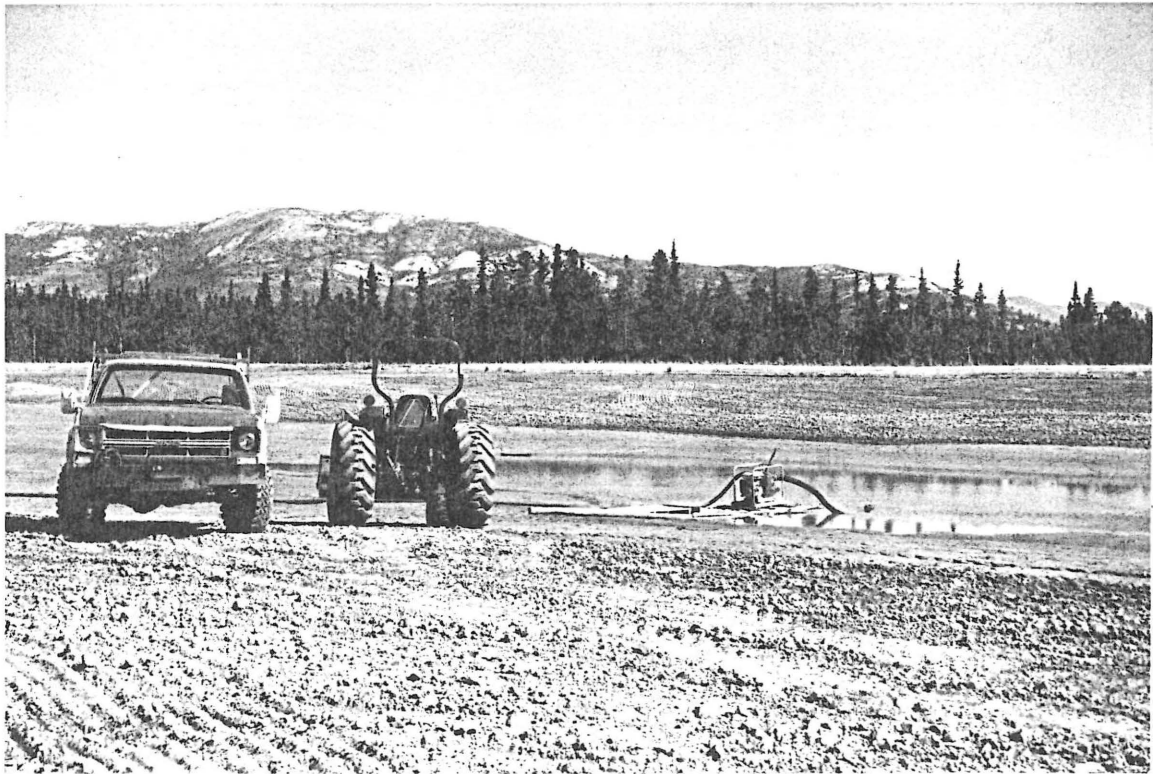
5. Equipment and temporary pond on tailings. David Craig photograph
