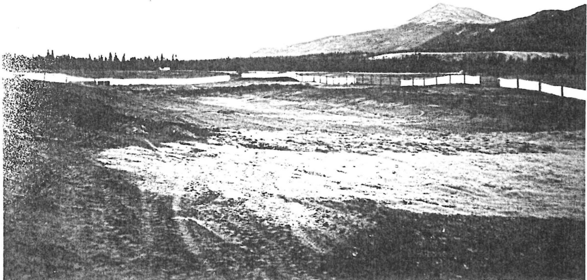
3. Sawdust (10 cm) on tailings.
